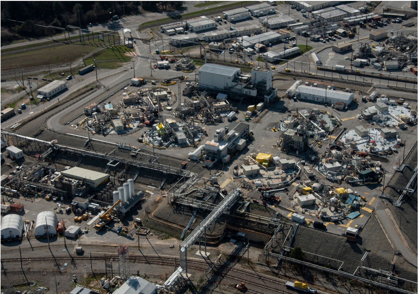
SRS has a total of 51 waste tanks built in the Site's F and H Areas; eight of those tanks have been operationally closed.
