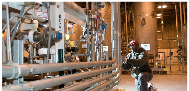
ETP is operated by personnel that are certified by the South Carolina Environmental Certification Board.
