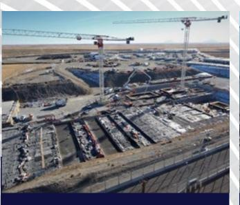
Began construction of the Naval Spent Fuel Handling Facility's massive concrete foundations with over 48,000 cubic yards of concrete placed to-date on bedrock.
