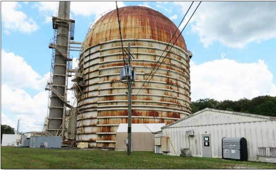
A view of the Experimental Gas-Cooled Reactor at Oak Ridge National Laboratory. The Oak Ridge Office of Environmental Management and cleanup contractor UCOR are set to fully deactivate the facility for eventual demolition.
