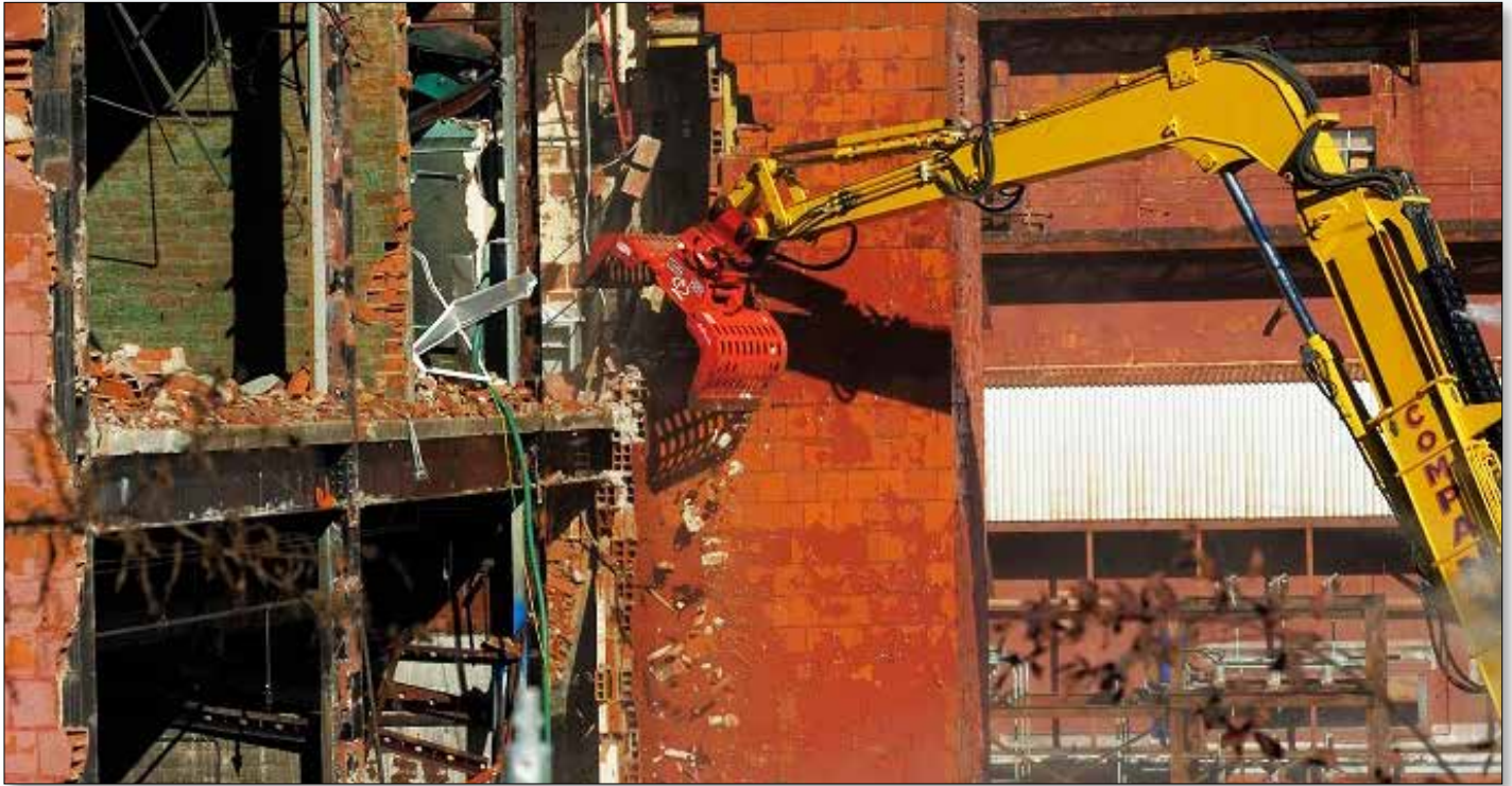
EM workers begin tearing down Building 9210 at Oak Ridge on November 16.
