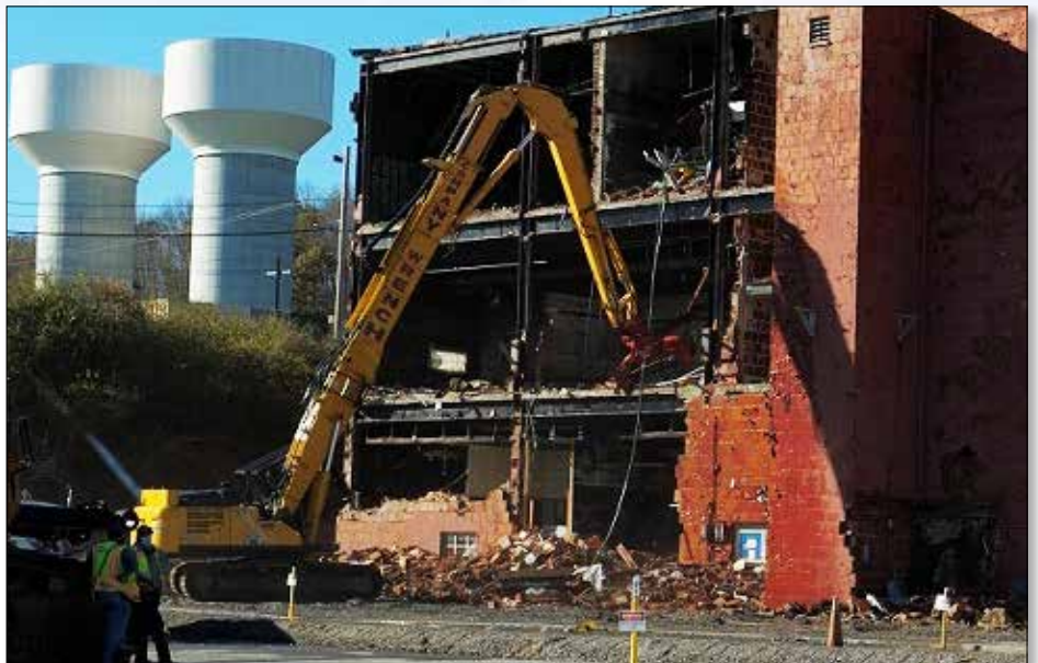
(Above) EM crews begin knocking down the three-story 65,000-square-foot Building 9210 at Y-12 National Security Complex on Nov. 16. (Below) A view of the conditions inside one of the remaining Biology Complex facilities, which date back to the 1940s. These buildings are part of Oak Ridge’s inventory of excess contaminated facilities to be addressed by cleanup workers.
