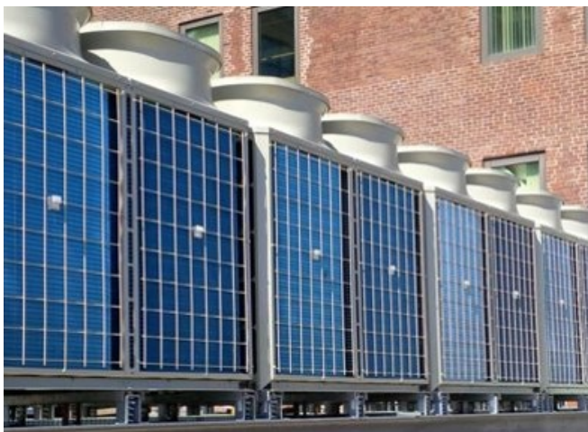
Variable refrigerant flow (VRF) units serve the space conditioning needs of large office buildings.
