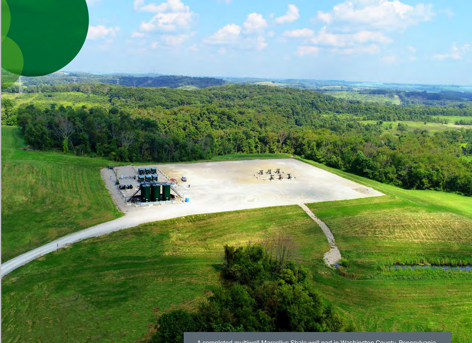
A completed multiwell Marcellus Shale well pad in Washington County, Pennsylvania.
