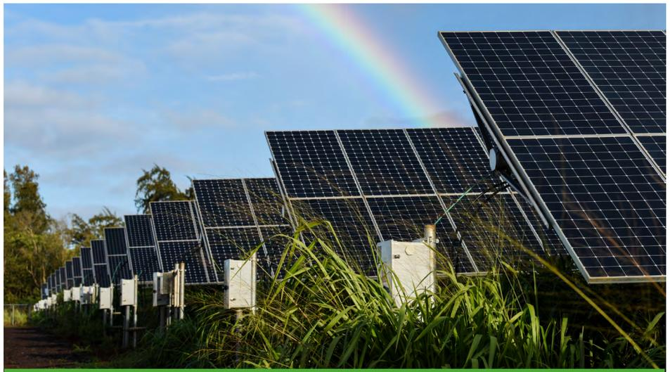
The AES Lawai Solar Project in Hawaii consists of a 28-megawatt solar photovoltaic system with a 100-megawatt-hour battery energy storage system. Photo courtesy of Dennis Schroeder / National Renewable Energy Laboratory.
