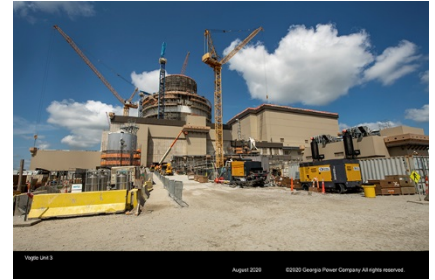
Vogtle Unit 3 (Courtesy of Georgia Power/ Southern Company, August 2020)
