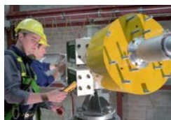
Photo by Warren Gretz, NREL 12420
