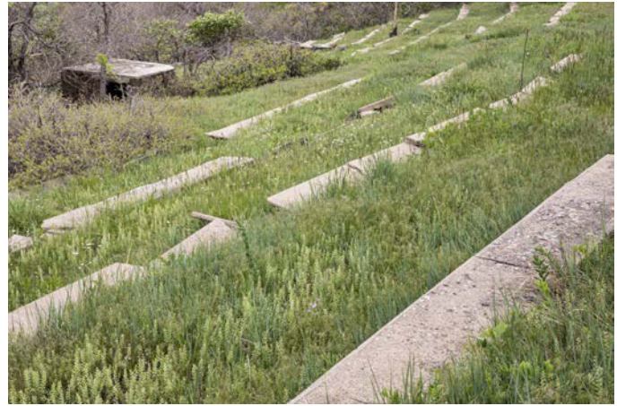
The Colorado Amphitheater, built in 1935, is a natural stone amphitheater that remains on the side of South Table Mountain, north of the STM Campus. The structure is listed on the National Register of Historic Places. Photo by Werner Slocum, NREL 56807
