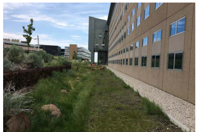
Surface water is conveyed through many drainageways on the STM Campus, including this grassy swale located north of the Research Support Facility (RSF). Photo by Brenna Birt, NREL 60727
