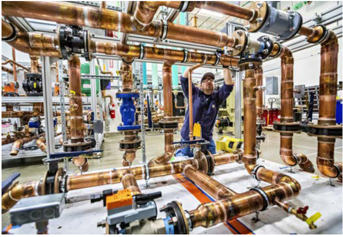
An NREL research technician works on finding ways for a commercial building to store energy to offset costs during peak hours, using both thermal and battery power at the Energy Systems Integration Facility (ESIF) at the STM Campus. Photo by Werner Slocum, NREL 60946
