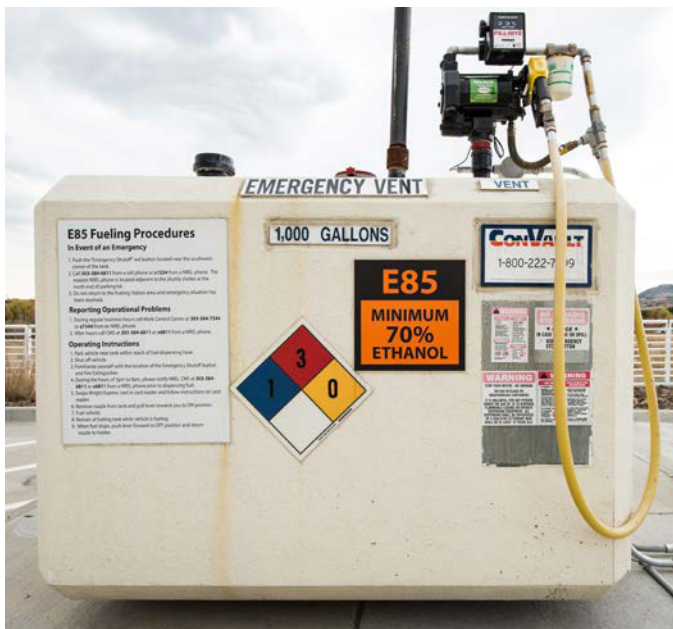
A 1,000-gallon gasoline aboveground storage tank (AST) on the STM Campus is maintained to refuel site support vehicles.
