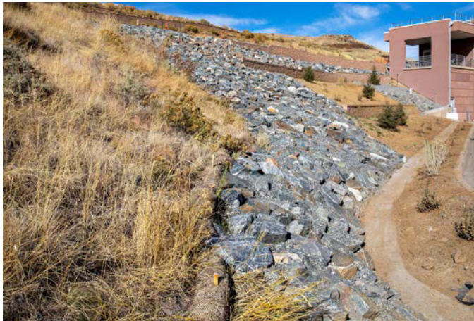
Significant progress was made in 2019 to stabilize the eroding hillside adjacent to the Field Test Laboratory Building (FTLB) at the STM Campus. Photo by Werner Slocum, NREL 61696
