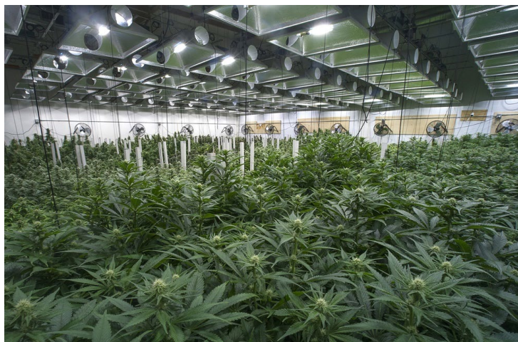
Figure 2-2 High Intensity Sole-Source Farm for Hemp. The grow area is fully indoors with no natural sunlight, and all light is provided by fixtures above the grow plane. [5]
