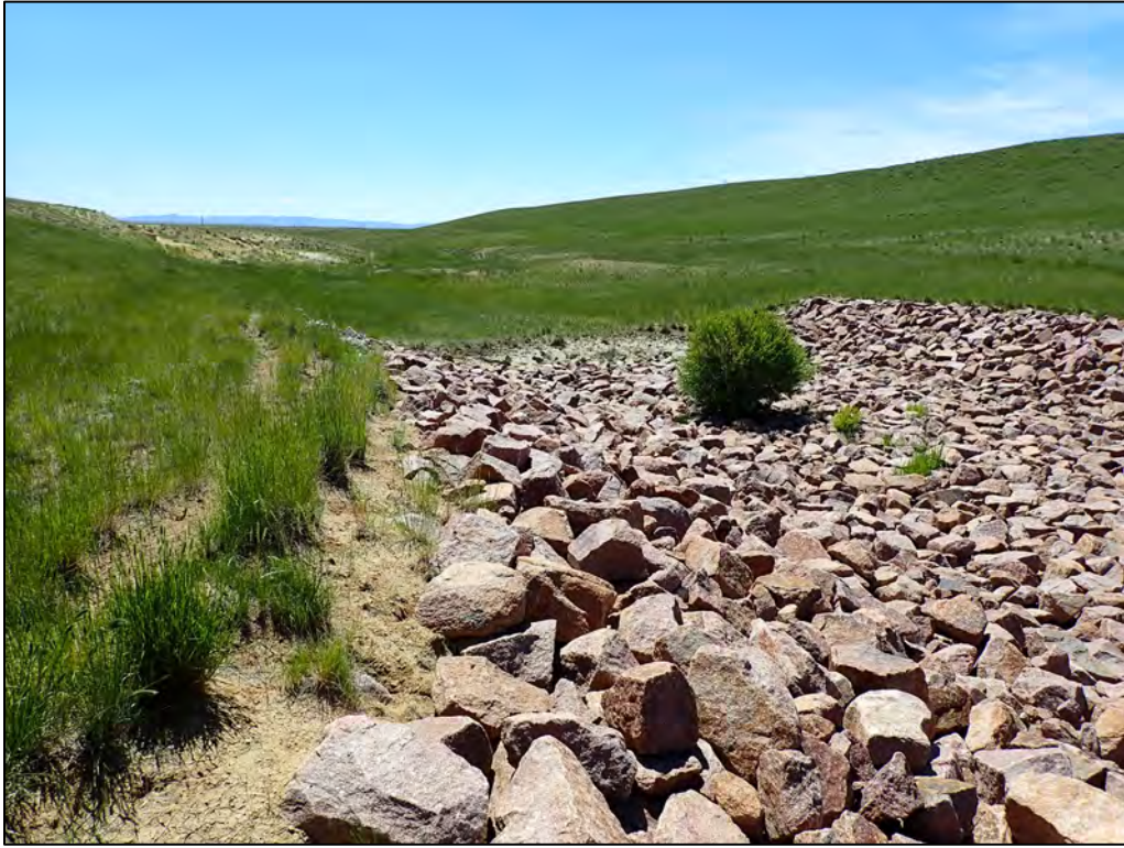
PL-13. Outlet of Riprap-Armored Diversion Channel
