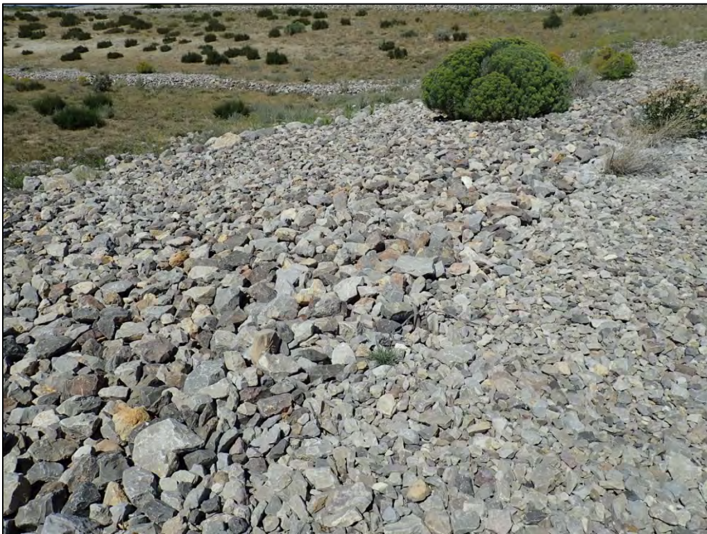
PL-12. Ancillary Cell West Side Slope with Small Depression on Cell Top Slope in Foreground
