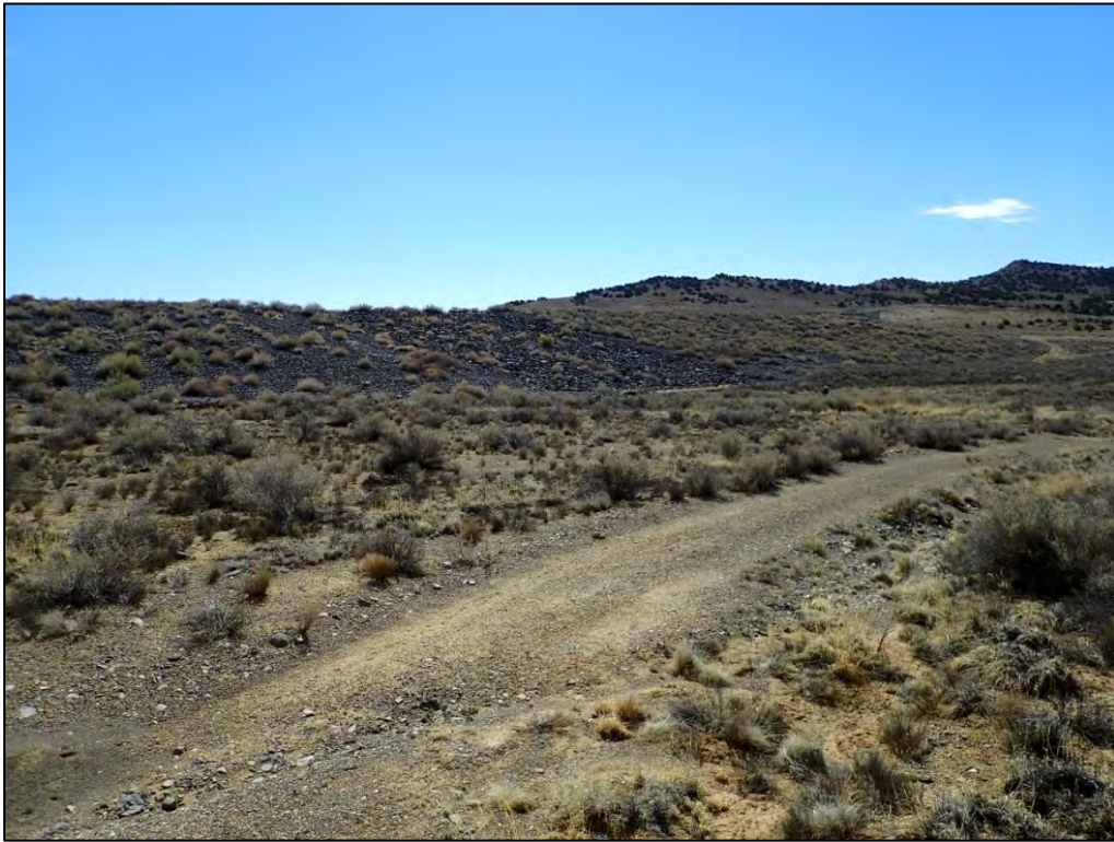
PL-9. Containment Dam Spillway
