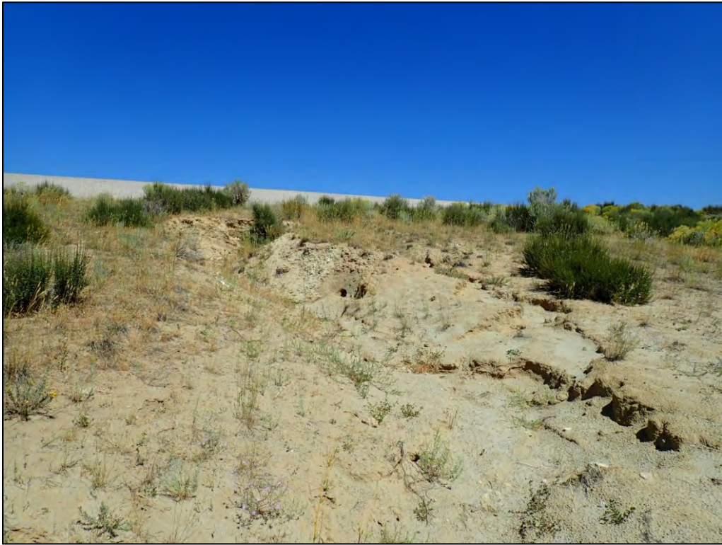
PL-19. Erosion West of Diversion Channel No. 2
