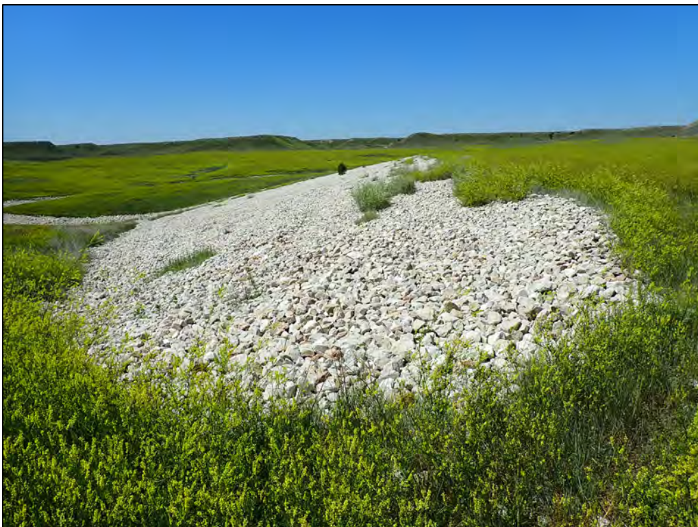
PL-8. East Portion of Containment Dam
