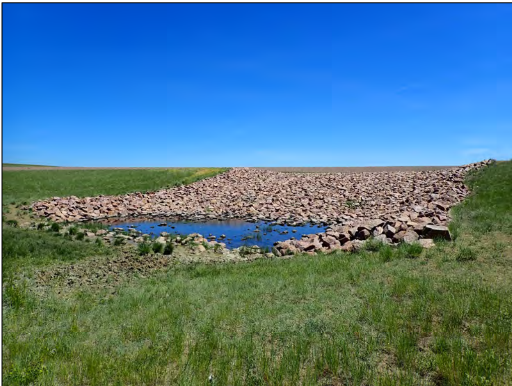
PL-8. North Swale Discharge Point (Runoff Present)
