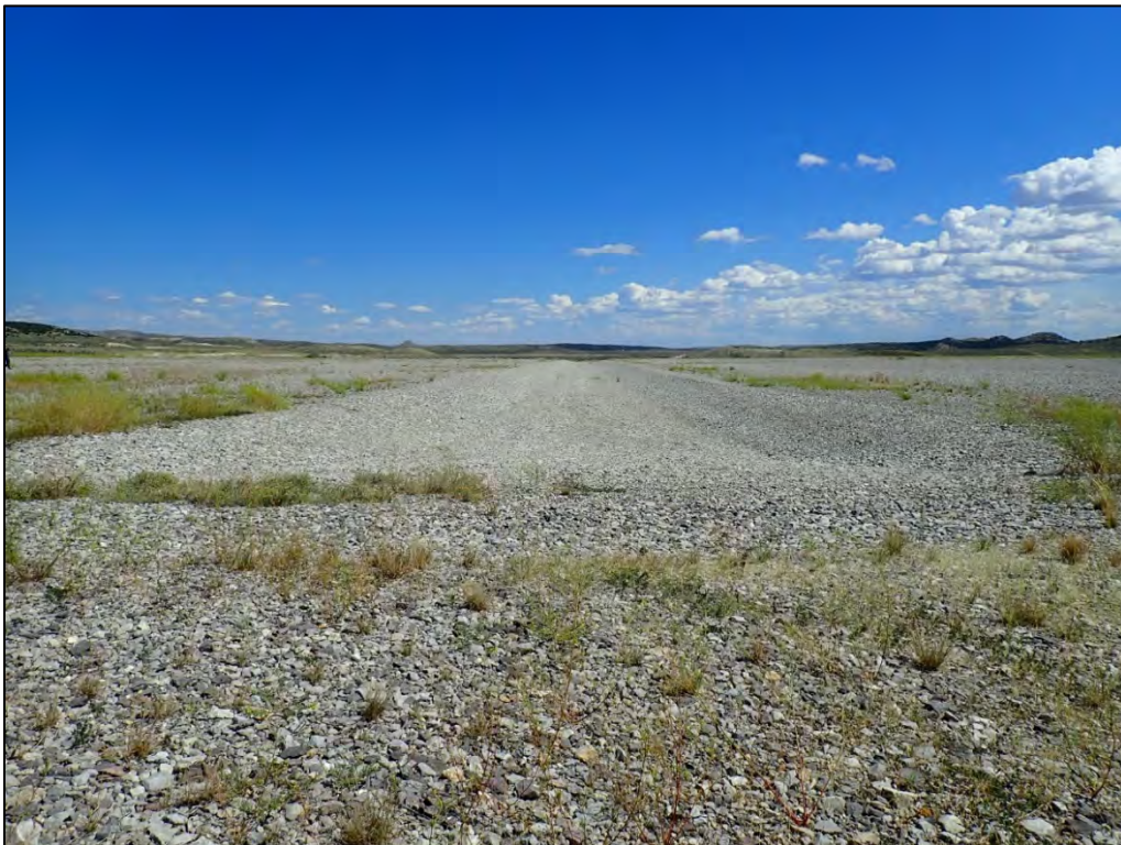
PL-8. Vegetation on Disposal Cell Top Slope and Diversion Channel No. 1
