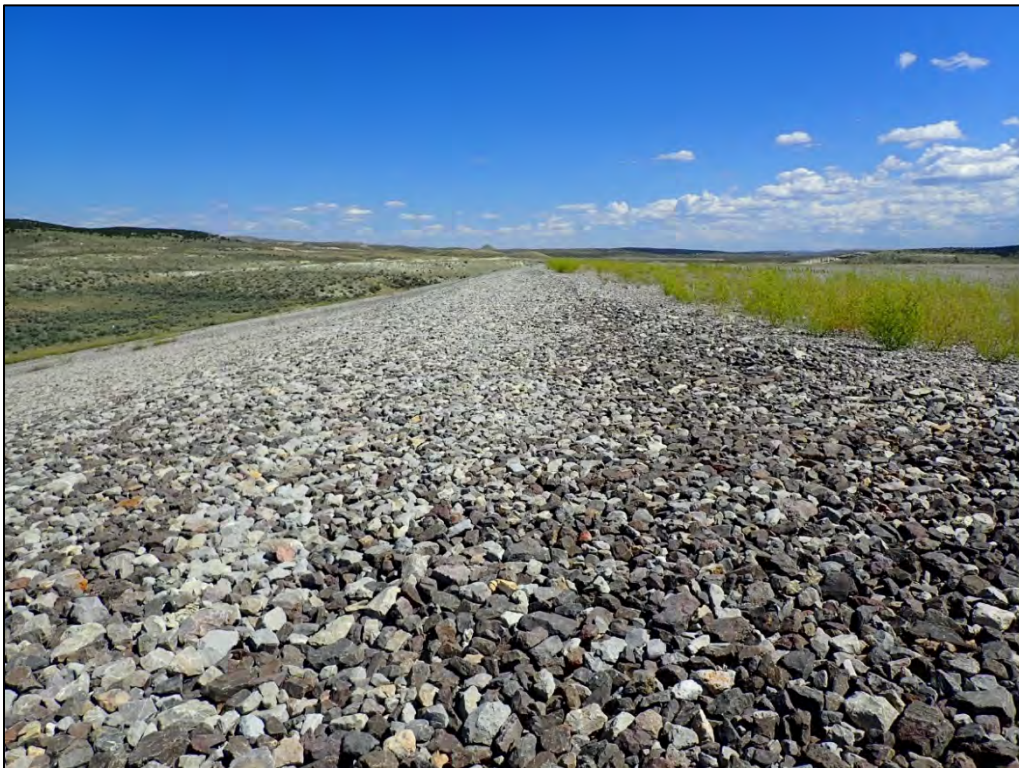
PL-10. Intersection of Disposal Cell Top Slope and North Side Slope
