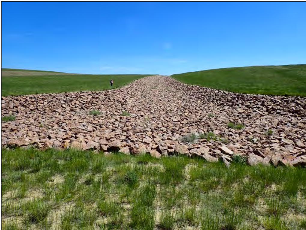
PL-12. Riprap-Armored Diversion Channel
