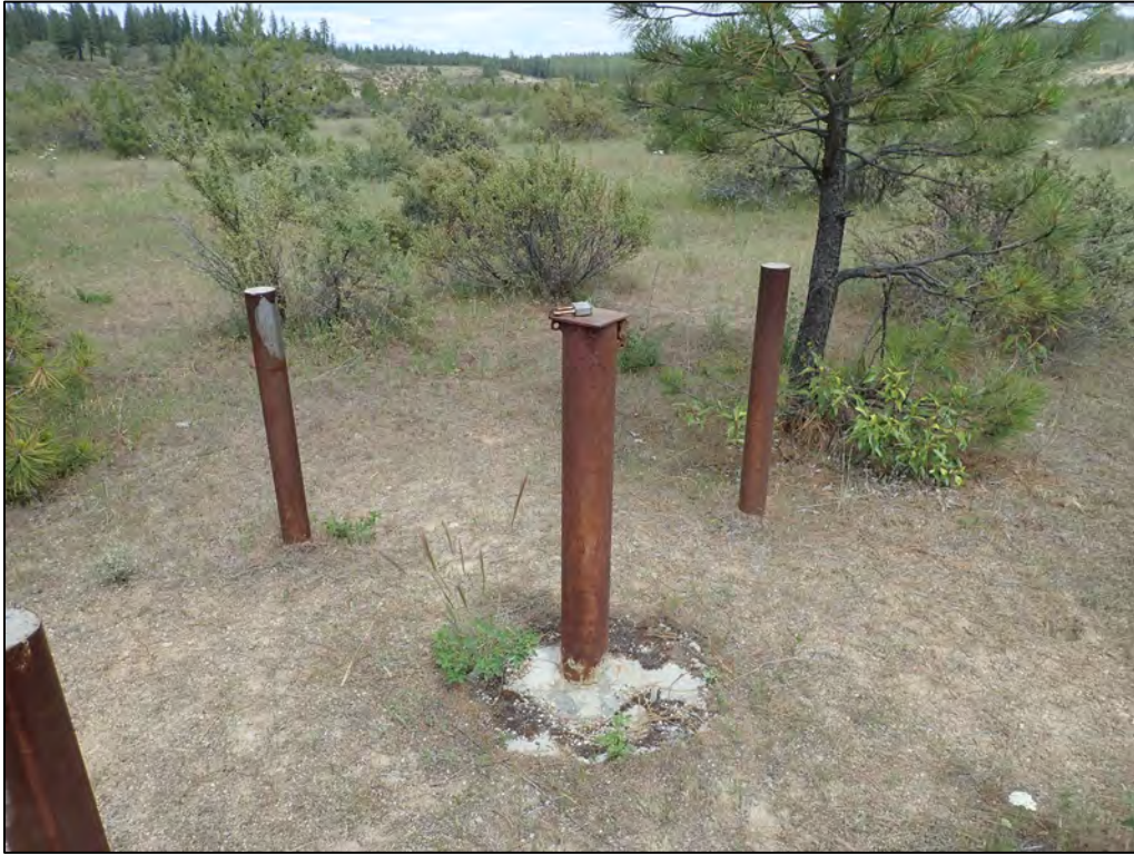
PL-5. Piezometer PZ-1
