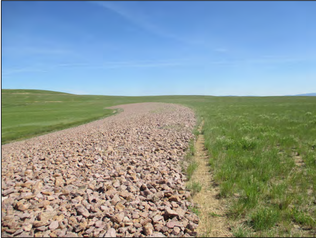
PL-7. Riprap-Armored Slope Between Upper Level and Lower Level of Disposal Cell
