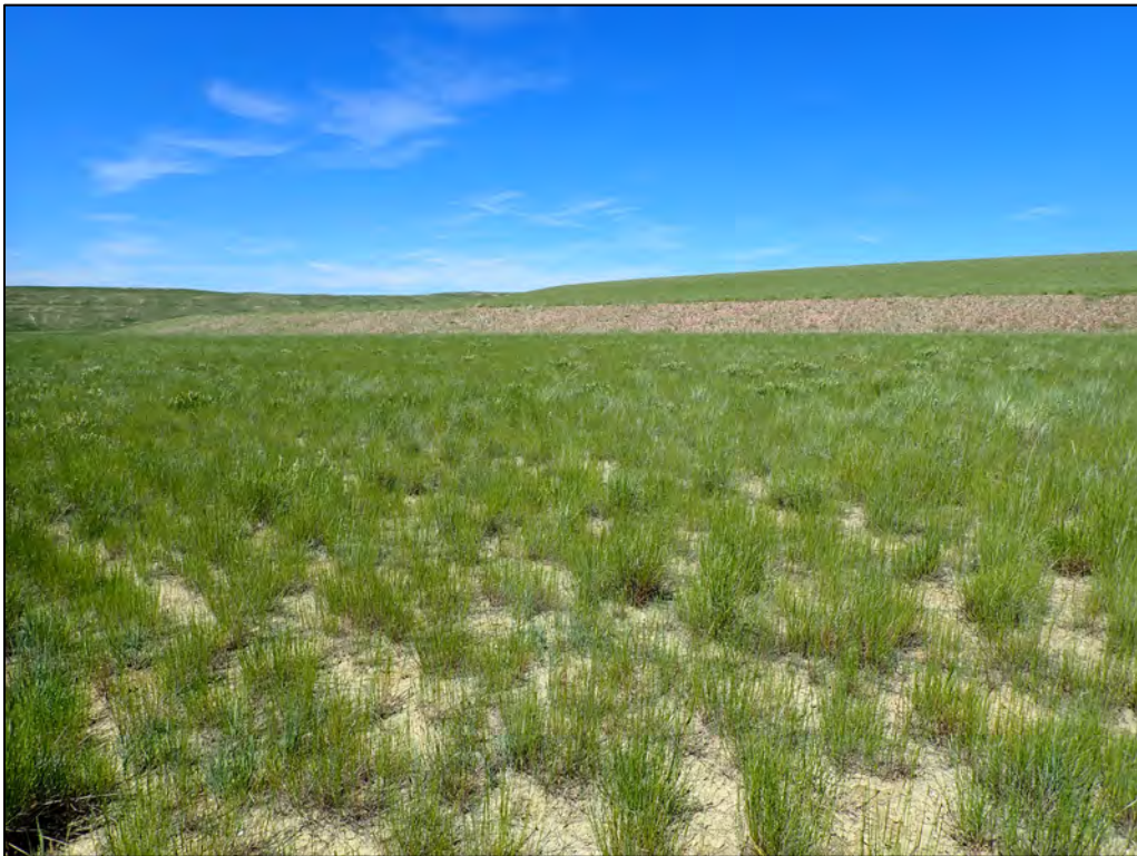
PL-10. Disposal Cell Dam Outslope
