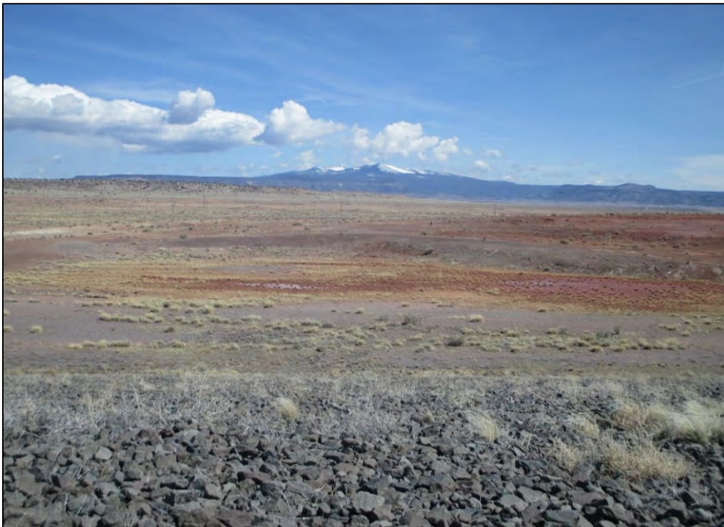
PL-18. East Side Slope of the Main Tailings Disposal Cell and Ephemeral Ponds (Wet)
