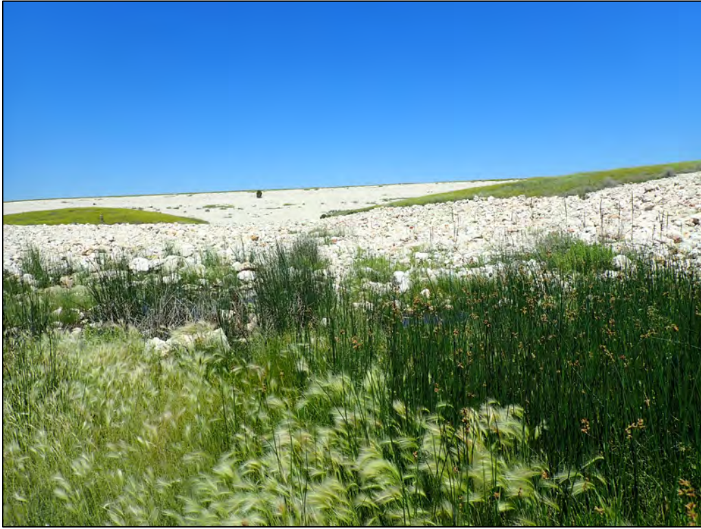
PL-11. Drainage Channel Outflow Area
