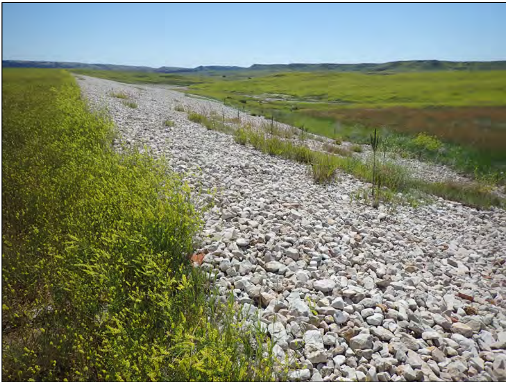
PL-6. West Portion of Containment Dam
