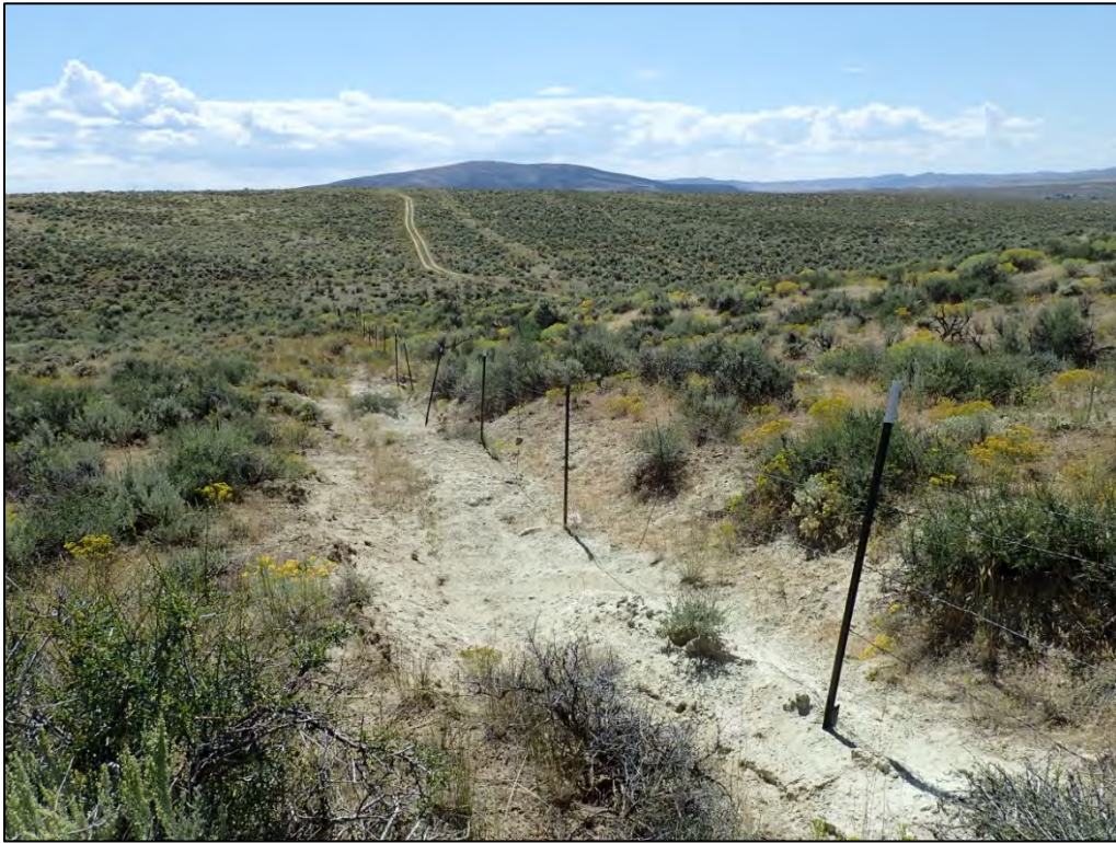
PL-1. Erosion Along Southwest Perimeter Fence
