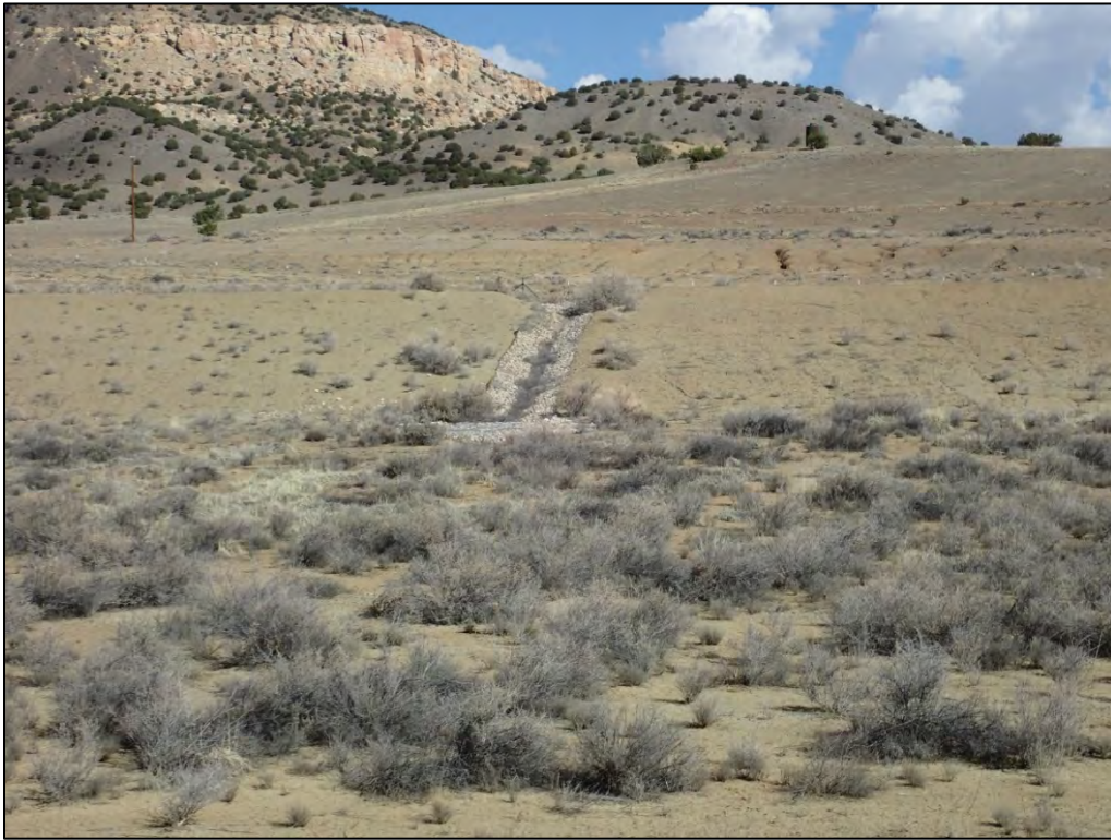
PL-13. Runoff Control Structure F
