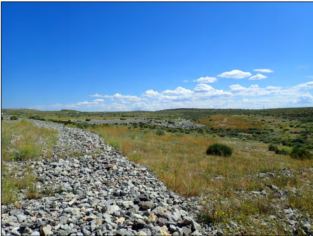
PL-18. Erosion Protection Rock Berm with Ancillary Cell and Diversion Channel No. 2 in Background
