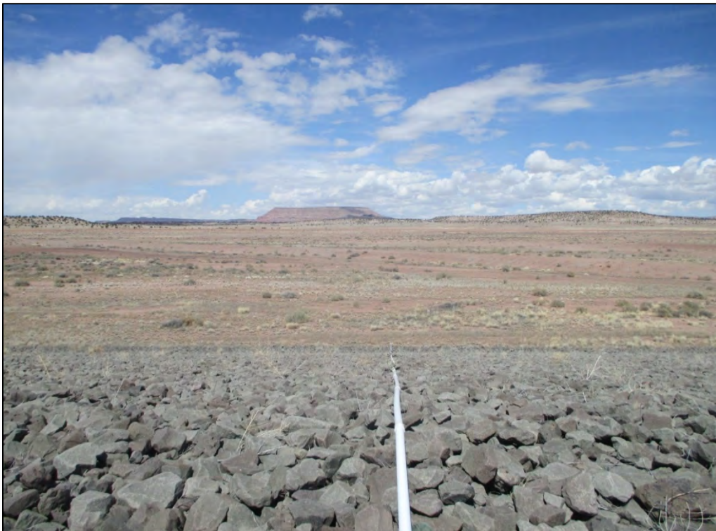
PL-8. Siphon on North Side Slope of the Main Tailings Disposal Cell
