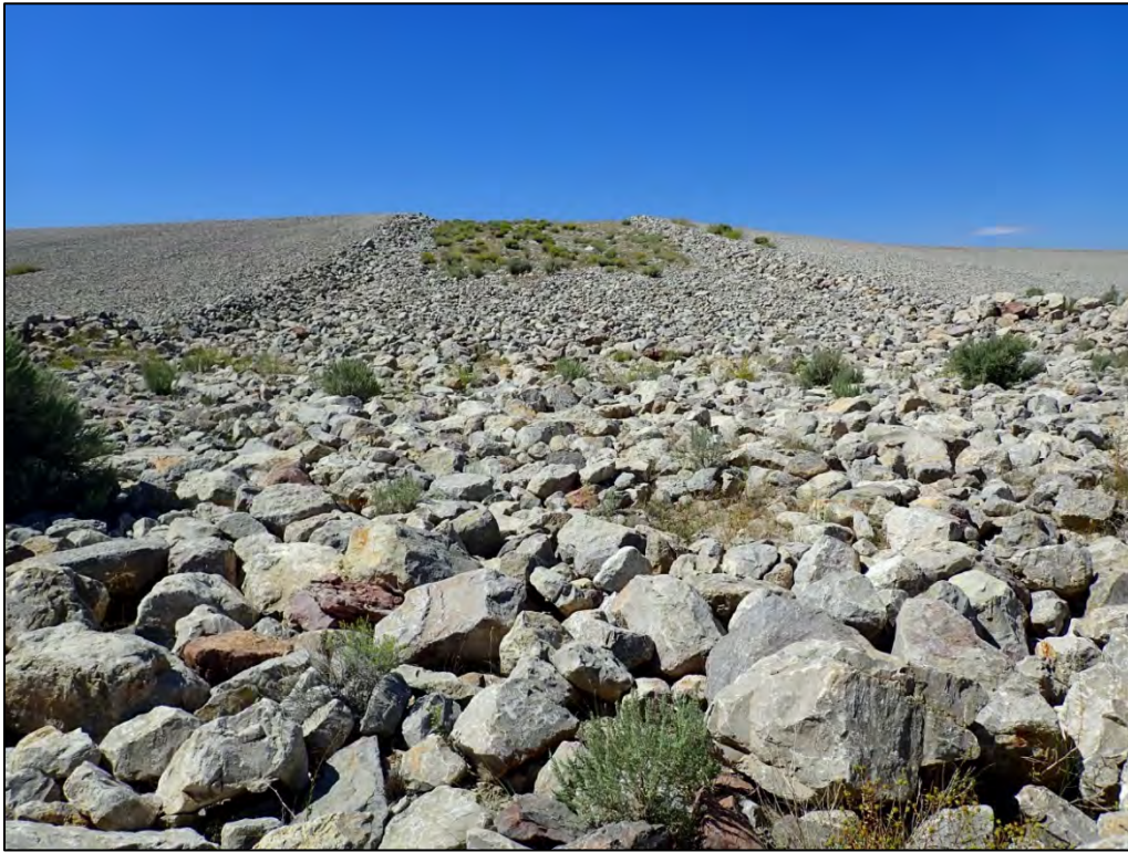
PL-15. Launch Rock Erosion Protection Basin on Disposal Cell East Side Slope
