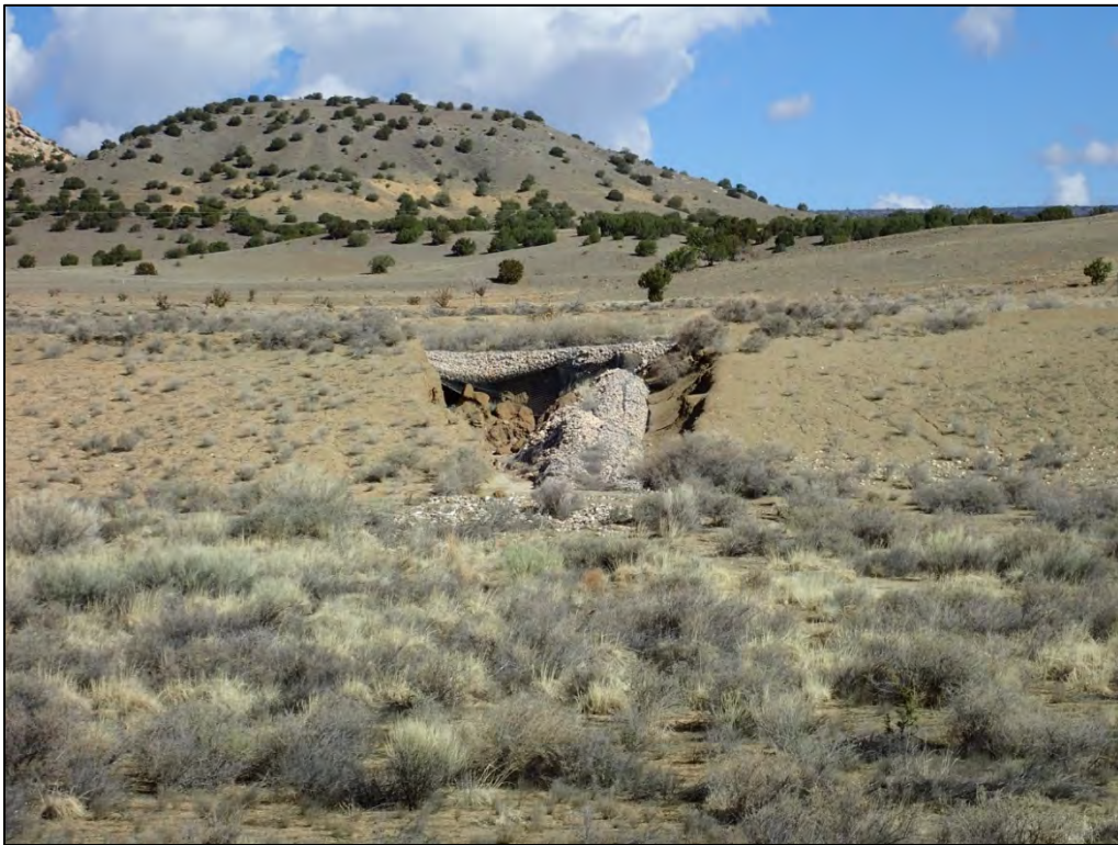
PL-14. Runoff Control Structure G
