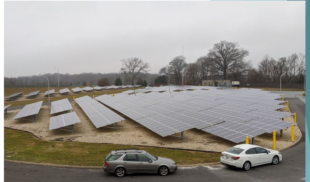
City of Wilmington (DE) Porter Treatment Plant $180,000 in annual savings from 2,288 ground-mounted solar panels that generate 650,000 kWh/year
