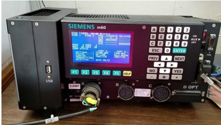
Figure II.1.2.8 A Siemens M60 controller used for traffic signal control in the city of Chattanooga
