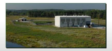
The aquifer cleanup, which involves pumping and treating water from the aquifer, is progressing as planned. Based on groundwater modeling, the aquifer cleanup is projected to be completed in 2026. To date, over 9.78 billion gallons of groundwater have been treated since 1993.
