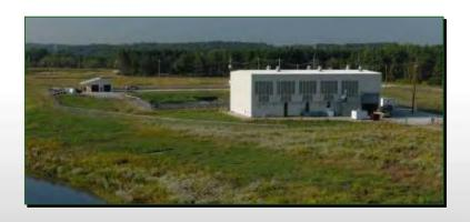
The aquifer cleanup, which involves pumping water from the aquifer and treating it, is progressing as planned. Groundwater modeling predicts that the aquifer cleanup will be completed in 2026. Since treatment began in 1993, approximately 28.9 billion gallons of groundwater have been pumped from the aquifer.
