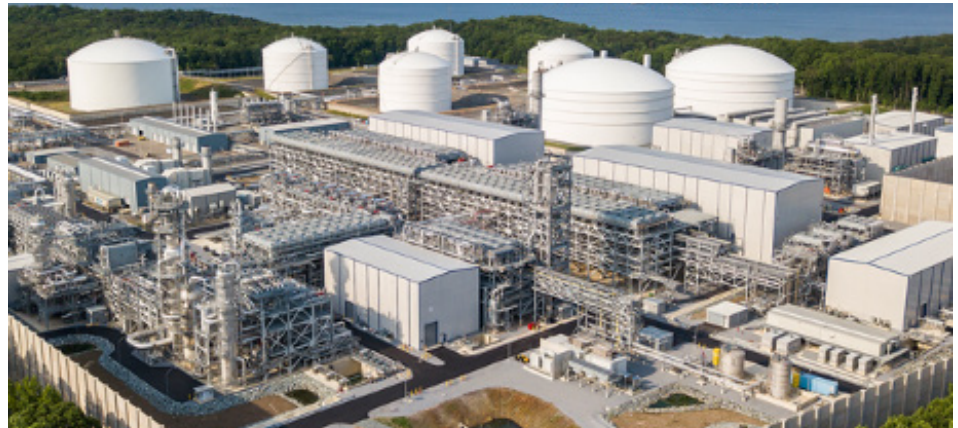
Image Source: Dominion Energy's Cove Point Liquefaction Plant in Lusby, MD.
