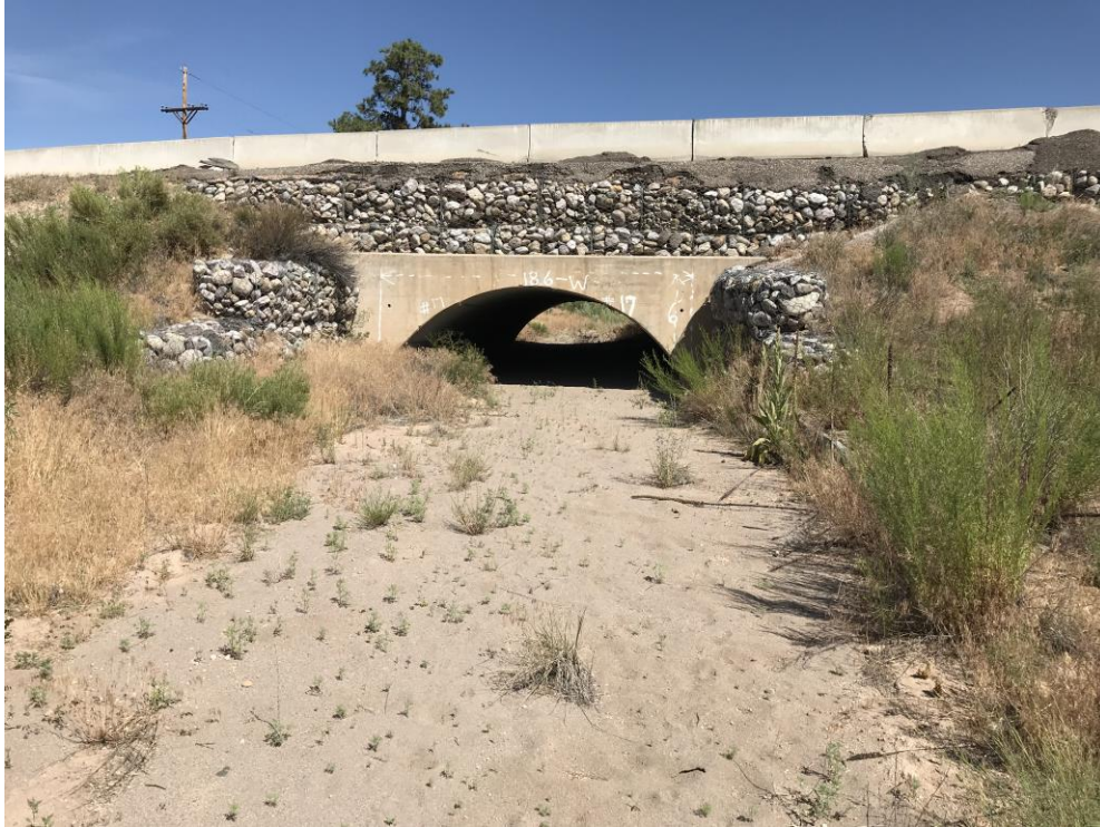
Photo 3. View of 18.25ft by 7.5ft multi-plate arch culvert under Ease Jemez Road, facing north. The culvert is partially filled with sediment.
