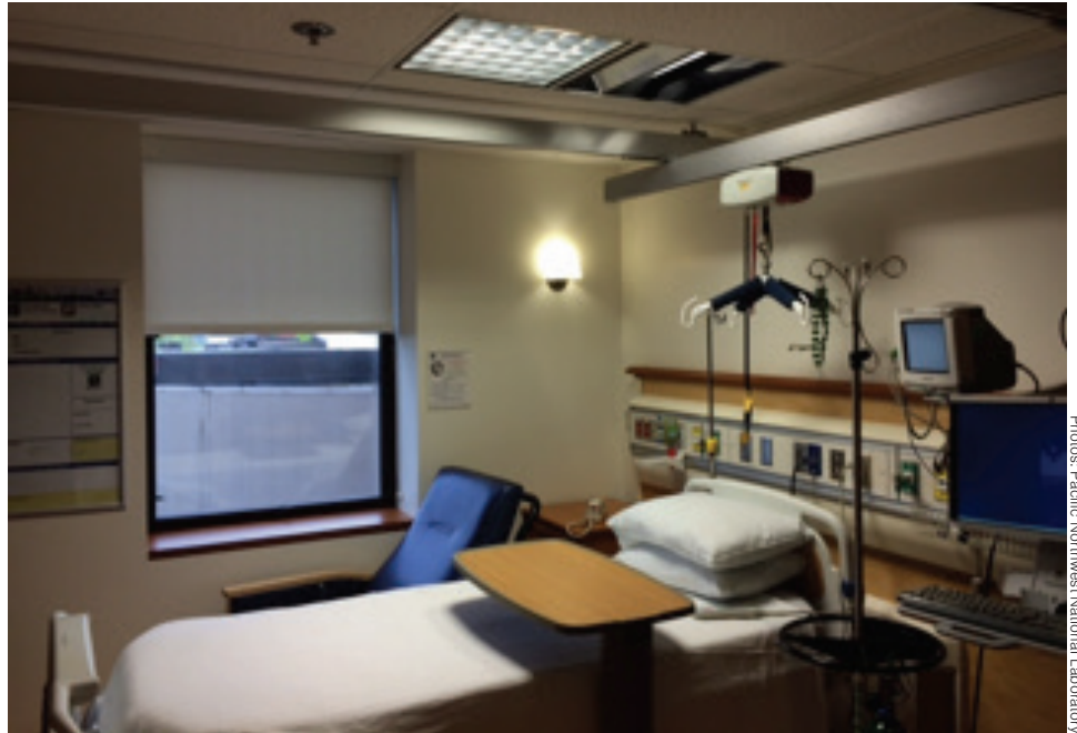
TEC patient room showing a multi-function recessed luminaire above the bed. For many years, this was the only luminaire in the room. A later upgrade added the wall sconce luminaire for the guest area.
