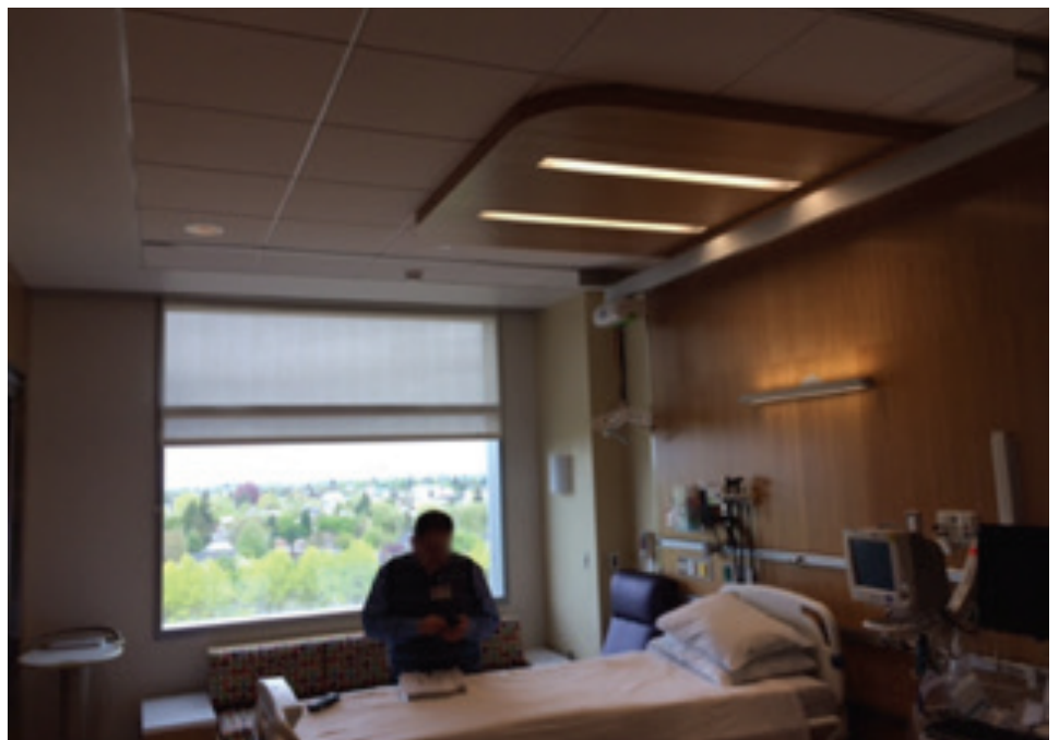
CEC patient room showing recessed round downlight luminaires for general room lighting, recessed linear luminaires over the bed for examinations, a wall-mounted linear luminaire for patient reading, and a wall sconce luminaire in the guest area.
