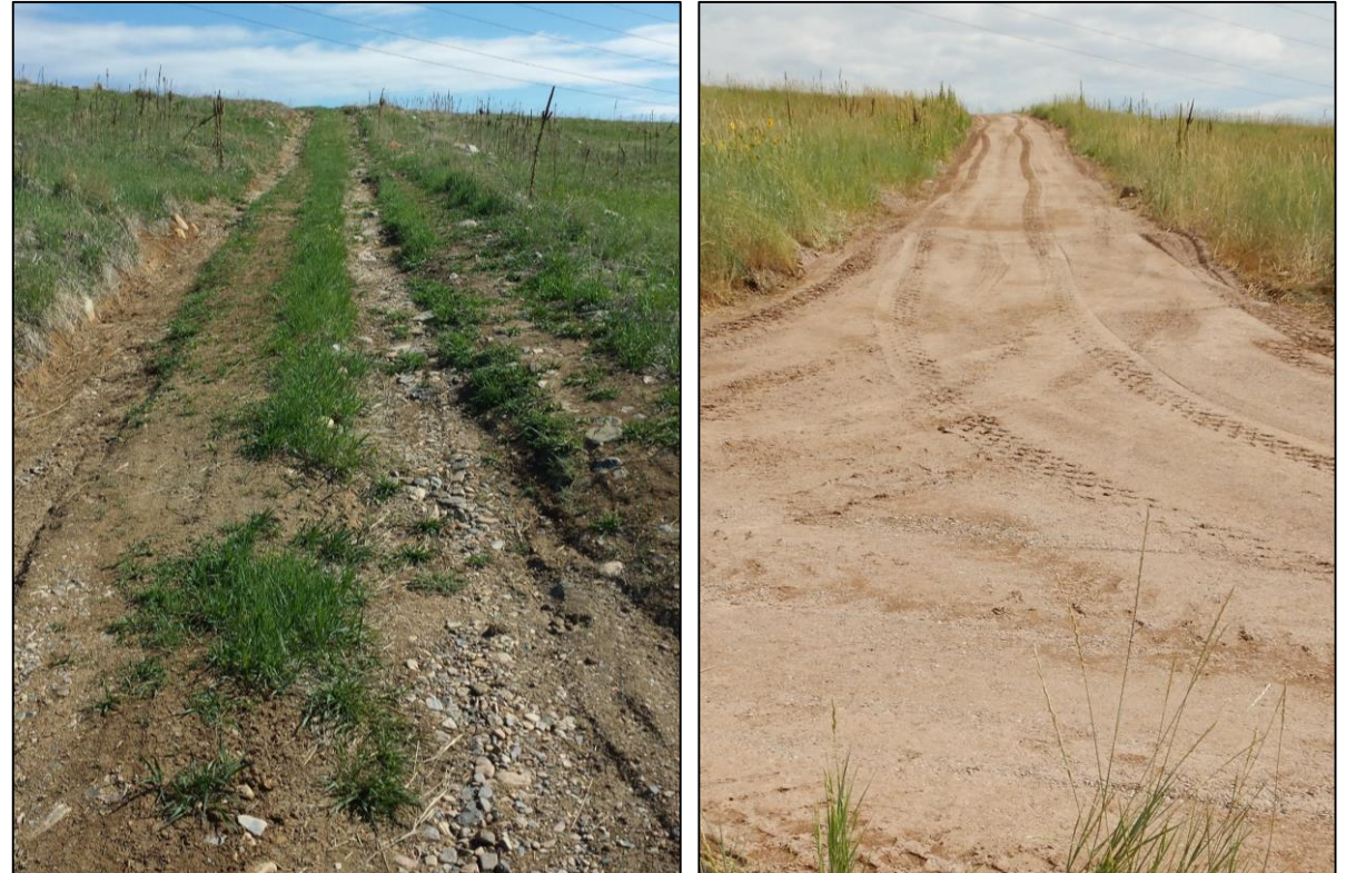
Road repairs — 2019 (before and after)
