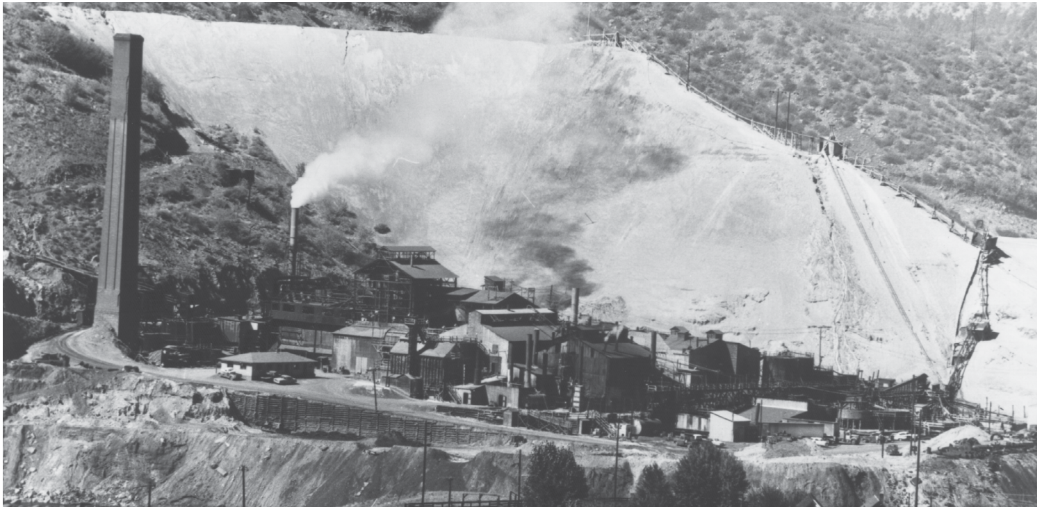
Durango mill during active operations (date unknown). The smokestack for the old lead smelter is to the left, with the large tailings pile and conveyances across the center.
