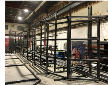
Steel Structure Being Built
