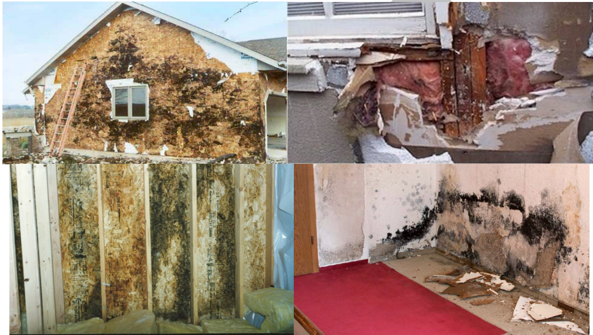
Figure 2-9: Examples of building envelope problems associated with extensive moisture intrusion. Photos (a) and (b) show the consequences of moisture intrusion and insufficient drying that has led to decay affecting multiple layers of the opaque envelope assembly. Photos (c) and (d) show the effect of moisture intrusion on the interior side of the opaque envelope. (Photos (a) and (b) courtesy of André Desjarlais, ORNL; photo (c) from the Building America Solution Center; photo (d) from the National Institute for Occupational Safety and Health)
