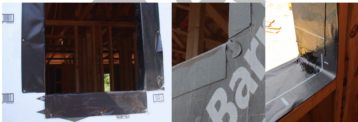
Figure 3-4: The corner of a roughed-out opening for a window in new residential construction is an example of the complex detailing required at interfaces to provide for air and water sealing. In (a), the air/moisture barrier has been wrapped around the window opening, but the corners have not been properly flashed, while in (b) and (c) the corners have been neatly detailed to ensure proper drainage around the window opening. The custom work required to accommodate each penetration through the facade creates a significant opportunity for errors and defects, which leads to variability in envelope performance from building to building. (Source: (a) EPA, (b, c) NIST)
