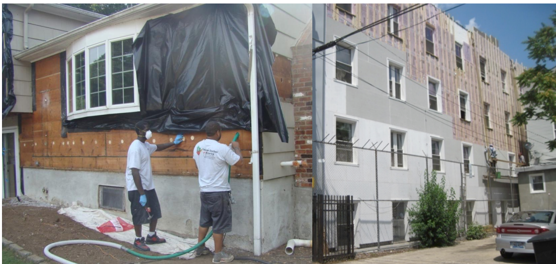
Figure 2-3: Drill-and-fill insulation (a) reduces heat transfer through walls by adding insulation to cavities between studs through small filling holes in each stud bay; overclad insulation retrofits (b) add one or more layers of insulation (typically rigid foam insulation) on top of the existing exterior facade; the layers are then covered by new exterior sheathing and finishing layers.
