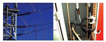
Mechanical devices are not the only sources of ultrasonic emission. Electrical equipment will also generate ultrasonic waves if arcing/tracking or corona are present.
