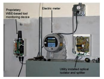
**Figure 8.9.1**. Installed wireless monitoring system for WBEbased system
