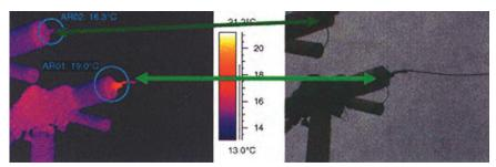
**Figure 6.2.4**. Air breaker problem. Highlighted by temperature difference between two different breakers. Likely caused by poor connection.
