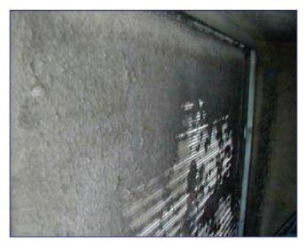
Figure 9.7.1. Cooling coil requiring cleaning
