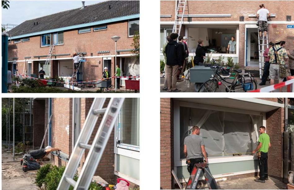
**Figure 8. Installation process images for RC Panels**
