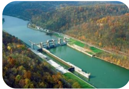
Non-Powered Dams and Conduits
