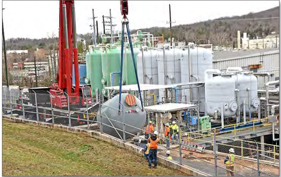
A crane lowers one of the five new vessels for a new modernized zeolite treatment system at Building 3608 at ORNL. It replaces an aging system in Building 3544.
