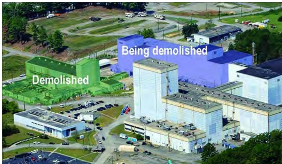
Workers are demolishing the K-1200 building of ETTP's Centrifuge Complex. The K-1004 lab was demolished earlier this year.
