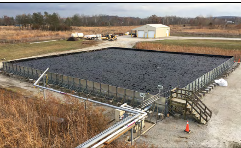
Top: Vegetation and aquatic plants growing in the backwash basin before refurbishment.
