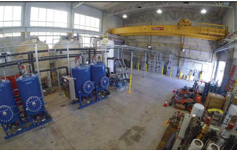
CAWWT tanks after right-sizing with a capacity of 50 gpm for current and future wastewater treatment needs.
