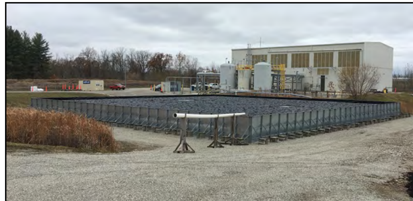
Top: CAWWT building and backwash basin before completion of the third and final phase of the wastewater treatment facility overhaul.
