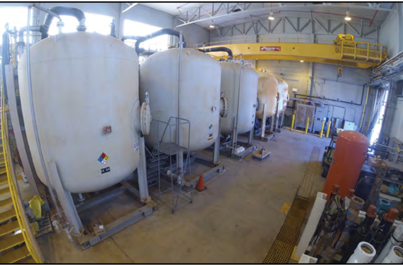
CAWWT tanks with a wastewater processing capacity of 1,800 gpm, built to support remediation era and initial post-closure wastewater treatment needs.
