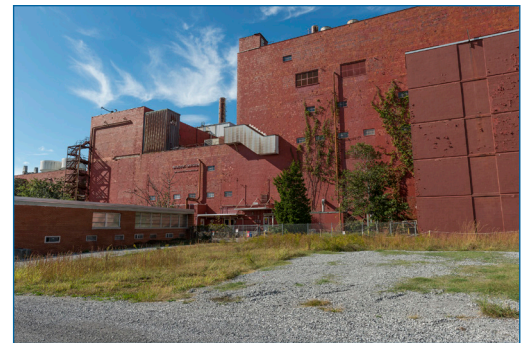
Demolition of the Biology Complex eliminates five high-risk buildings
