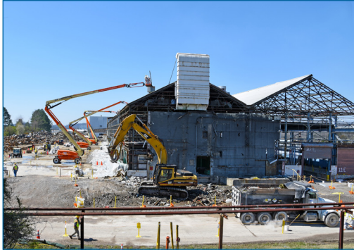
Demolition of Building K-1037
