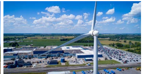
Photo courtesy of Hank Doster, One Energy Enterprise, LLC
