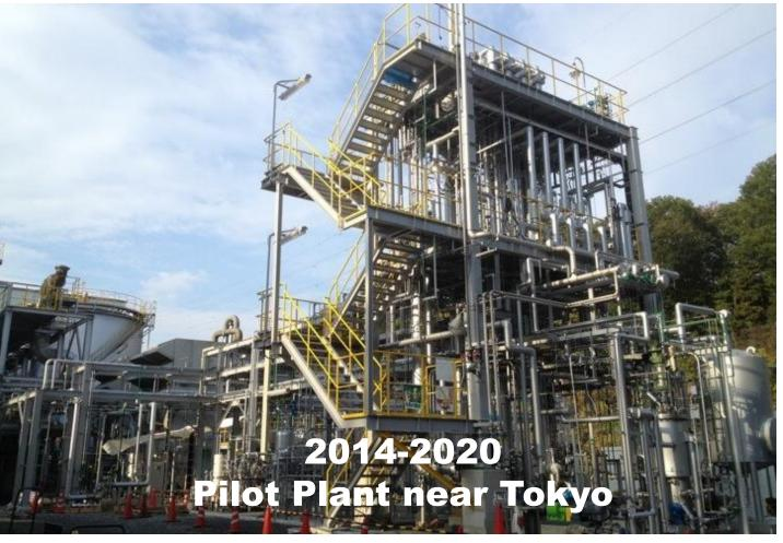
World-first demonstration of continuous direct ethanol production from MSW-derived syngas
