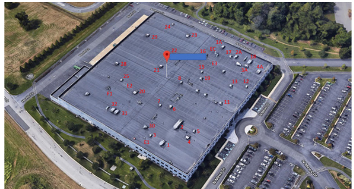
Based on a comprehensive evaluation of RTU fan consumption, current continuous fan operation results in consumption of a little over 1,000,000 kilowatt hours per year, almost 20% of the facility's electric bill. By placing the RTUs in fan-automatic mode during unoccupied time, the facility should save nearly $32,500 per year in electricity costs.
