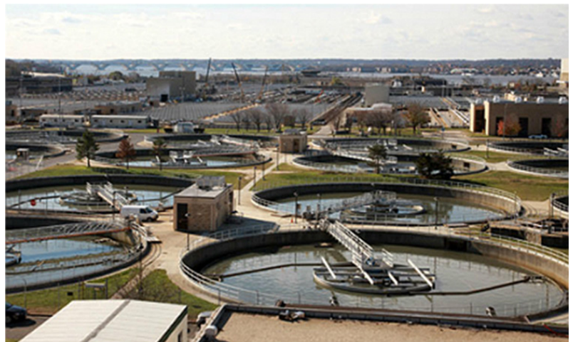
Blue Plains Advanced Water Resource Recovery Facility, Washington, D.C.
