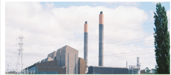
Facility Flexibility, Efficiency, and Value Enhancement
