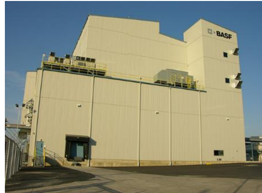
BASF's NMC battery materials plant in Elyria, Ohio
