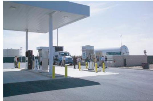
A liquid and compressed natural gas fueling station in Fresno, California.
