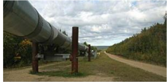
Pipelines are a common component of oil and gas infrastructure and are one element tracked in the GOGI database
