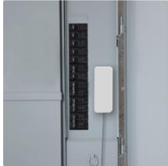
DIY Home Energy Monitoring Sensor installed and operational.
