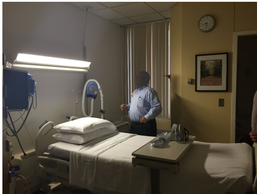
Figure A6: Hospital C patient room showing the wall-mounted luminaire with a hinged uplight section. The uplight section is in the examination position, directing its light toward the patient bed. The wall-mounted luminaire is the only electric lighting in the room.
