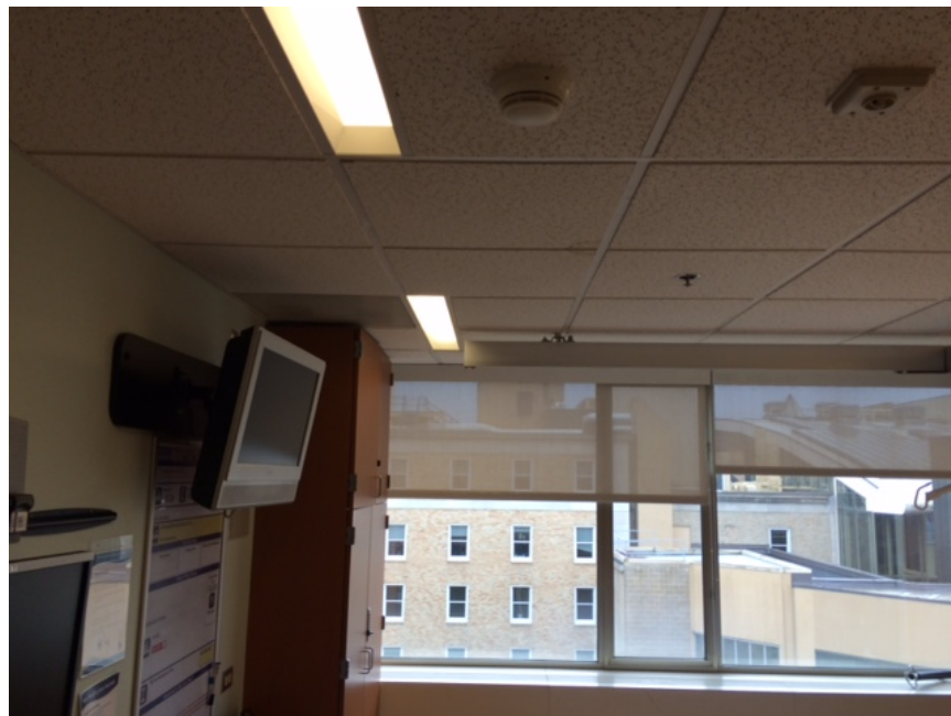
Figure A2: Hospital A patient room showing the recessed linear luminaires providing general room lighting.
