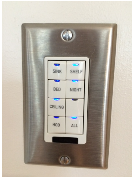
Figure A9: Hospital D patient room push-button lighting controller. HOB refers to the “head of bed” wall-mounted luminaire while “BED” refers to the recessed ceiling lighting over the bed. “CEILING” refers to the recessed downlight luminaires providing general room lighting.
