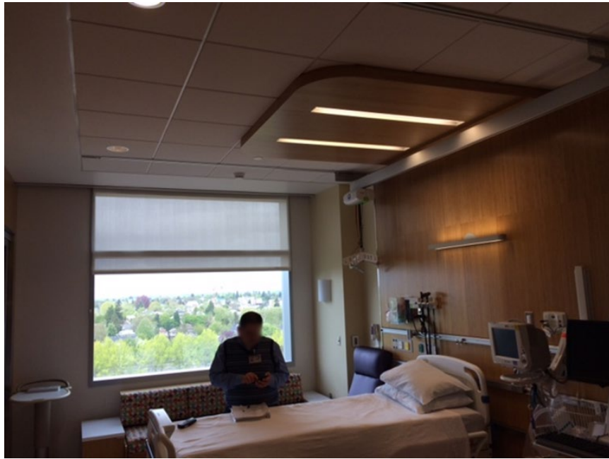
Figure A7: Hospital D patient room showing the recessed round downlight luminaires for general room lighting, the recessed linear luminaires over the bed, the wall-mounted linear luminaire for patient reading, and the wall sconce luminaire in the guest area.
