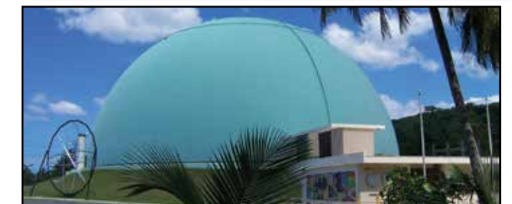
The decommissioned Boiling Nuclear Superheater reactor in Puerto Rico.
