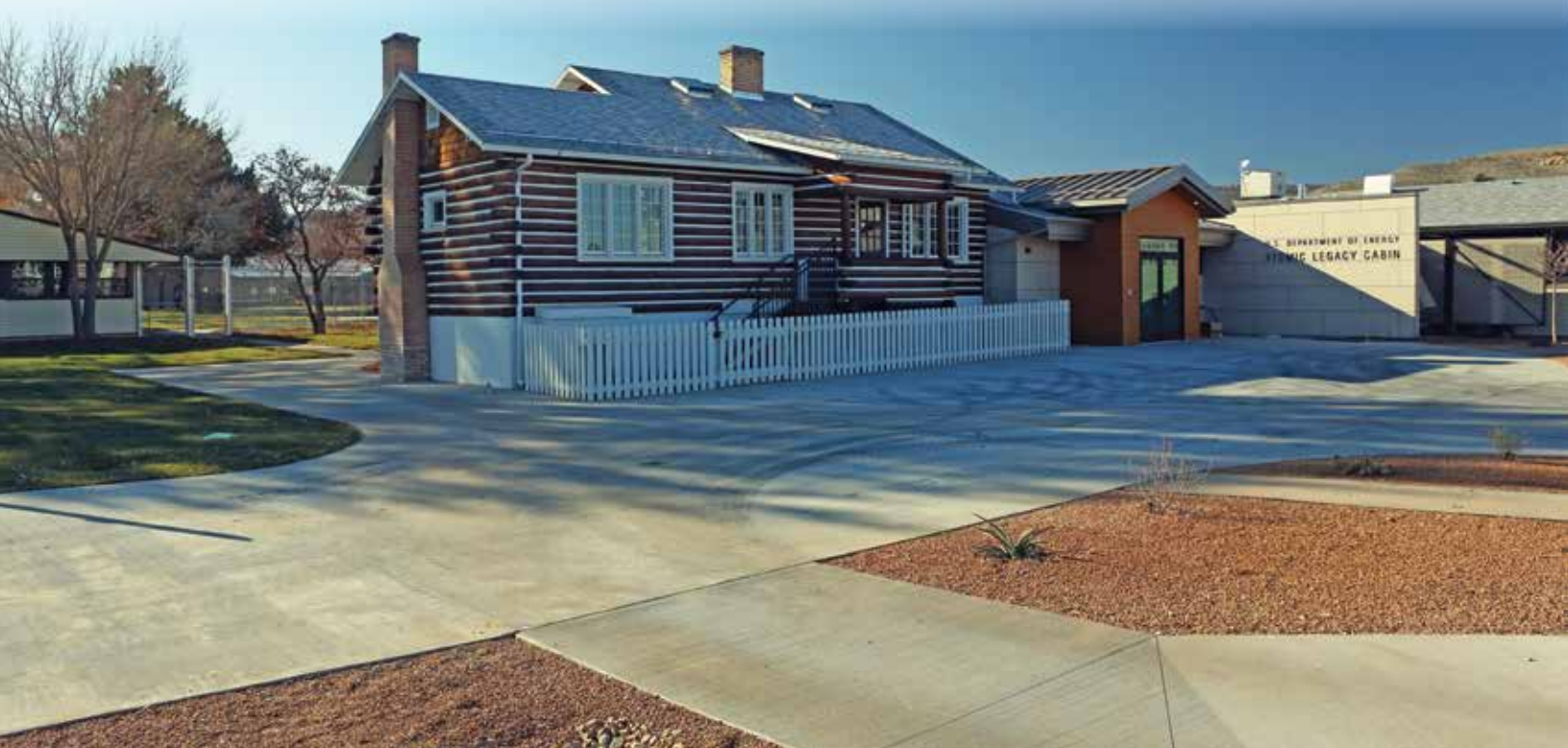
Atomic Legacy Cabin at the Grand Junction, Colorado, Site.
