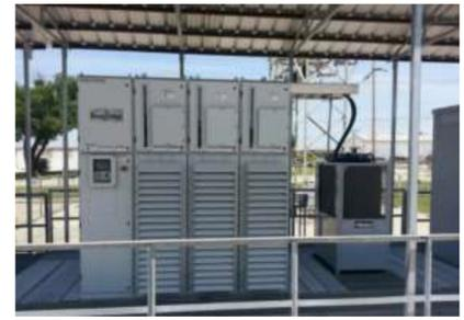
Left: Schematic view of an existing TECO-Westinghouse VersaBridge power converter module system with cabinet that houses the mains controller and three slice cabinets; each cabinet includes three power cubes, an isolation transformer, and slice controllers for the output and active front end controls. Right: A physical installation of a VersaBridge system. *Photo credit TECO-Westinghouse Motor Company.*
