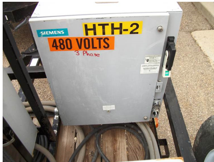
Figure 4. Typical Disconnect Switch
