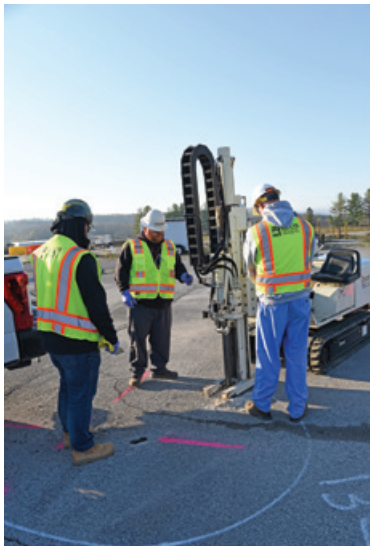
Workers sample the K-1232 slab after demolition
