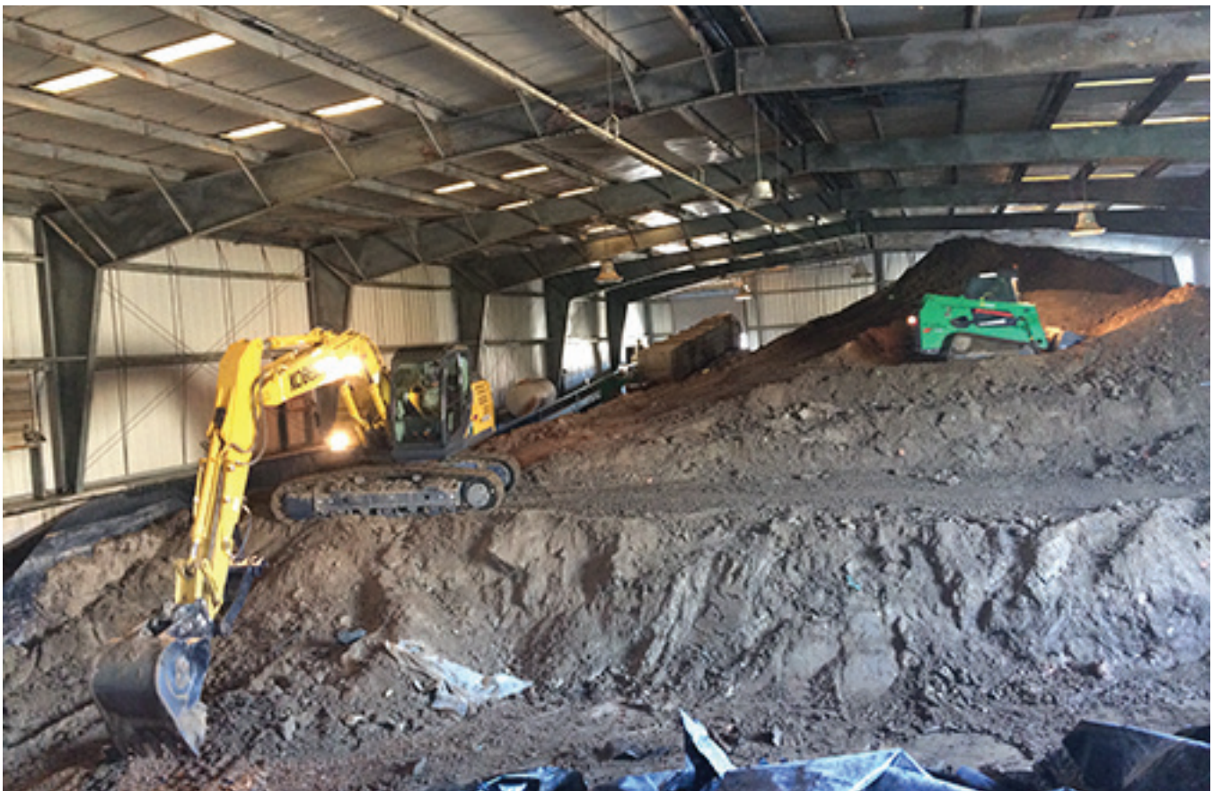
Workers dispose soil resulting from the closure of oil retention ponds
