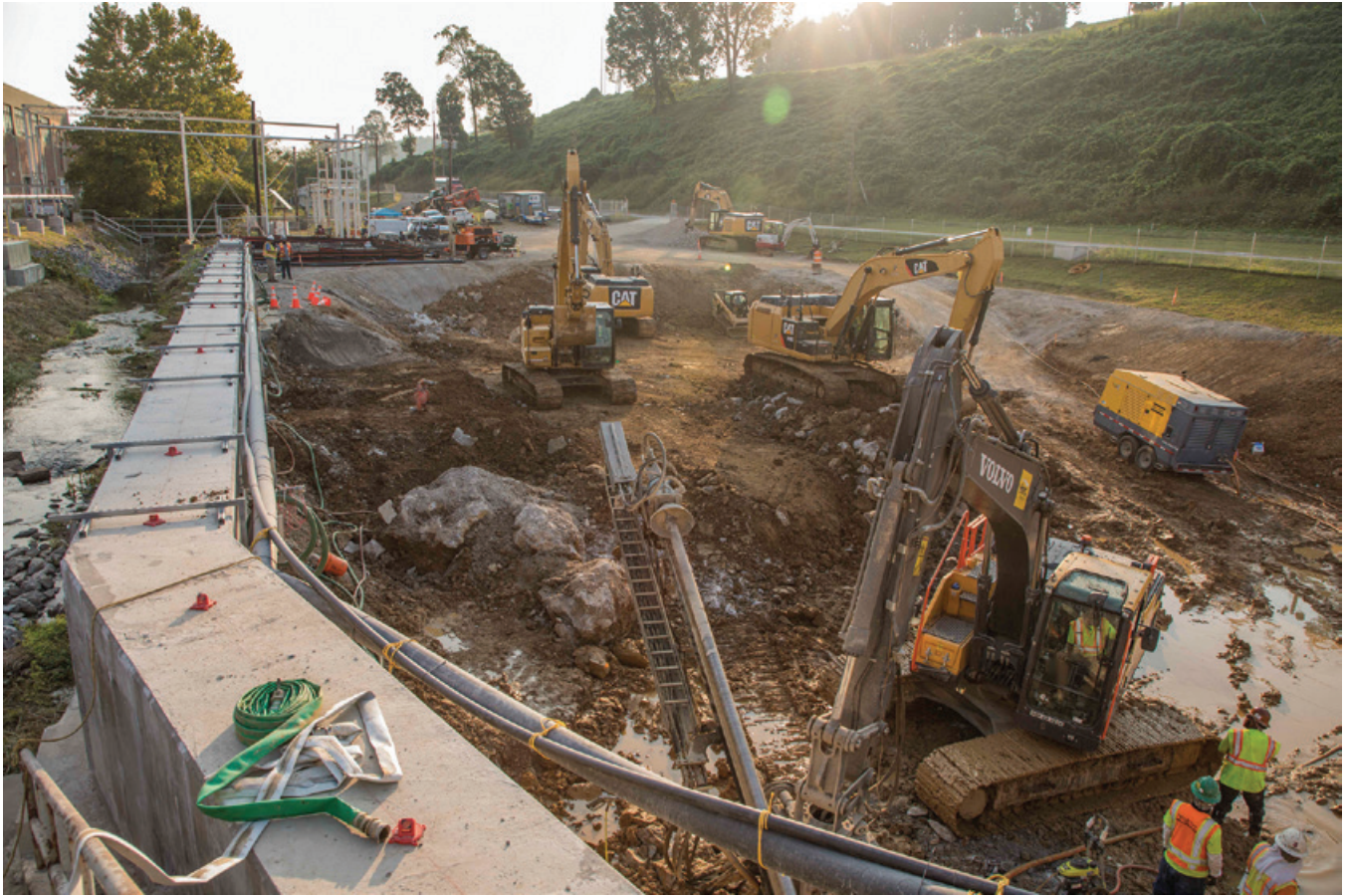
Excavation underway at the headworks facility area
