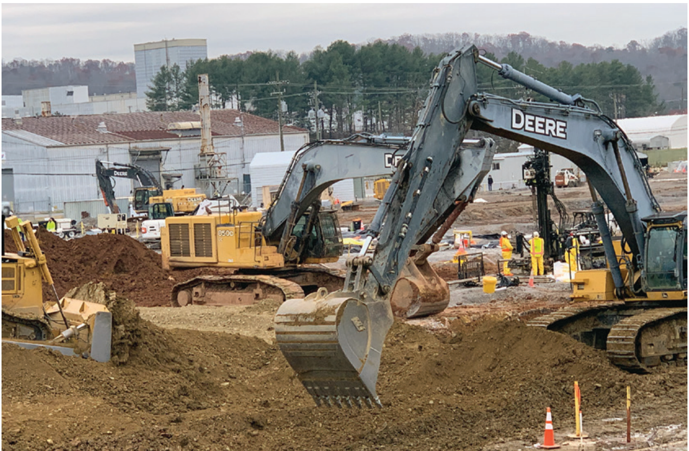
Excavation of Tc-99 contaminated soil
