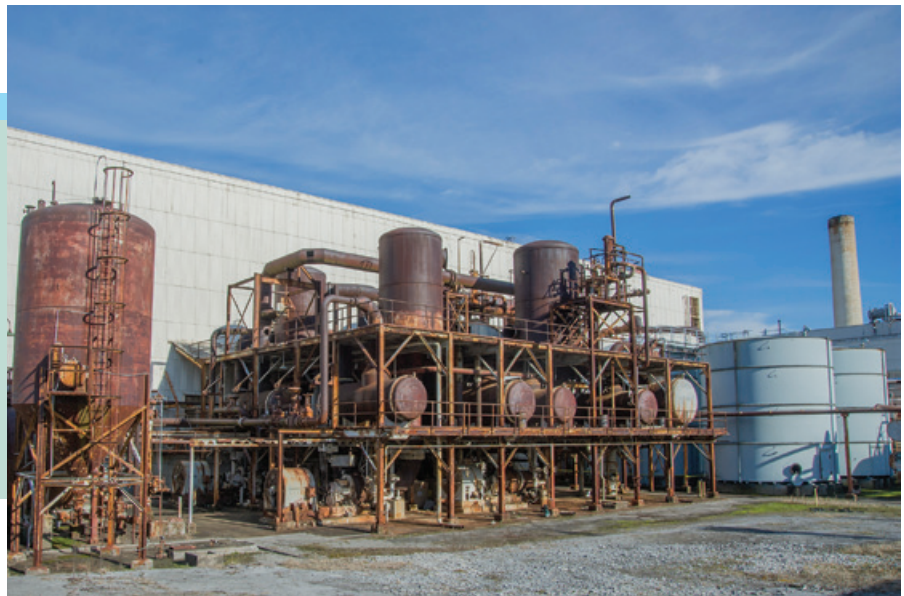
The West COLEX equipment before and after demolition. Below a worker is tapping and draining a pipe.
