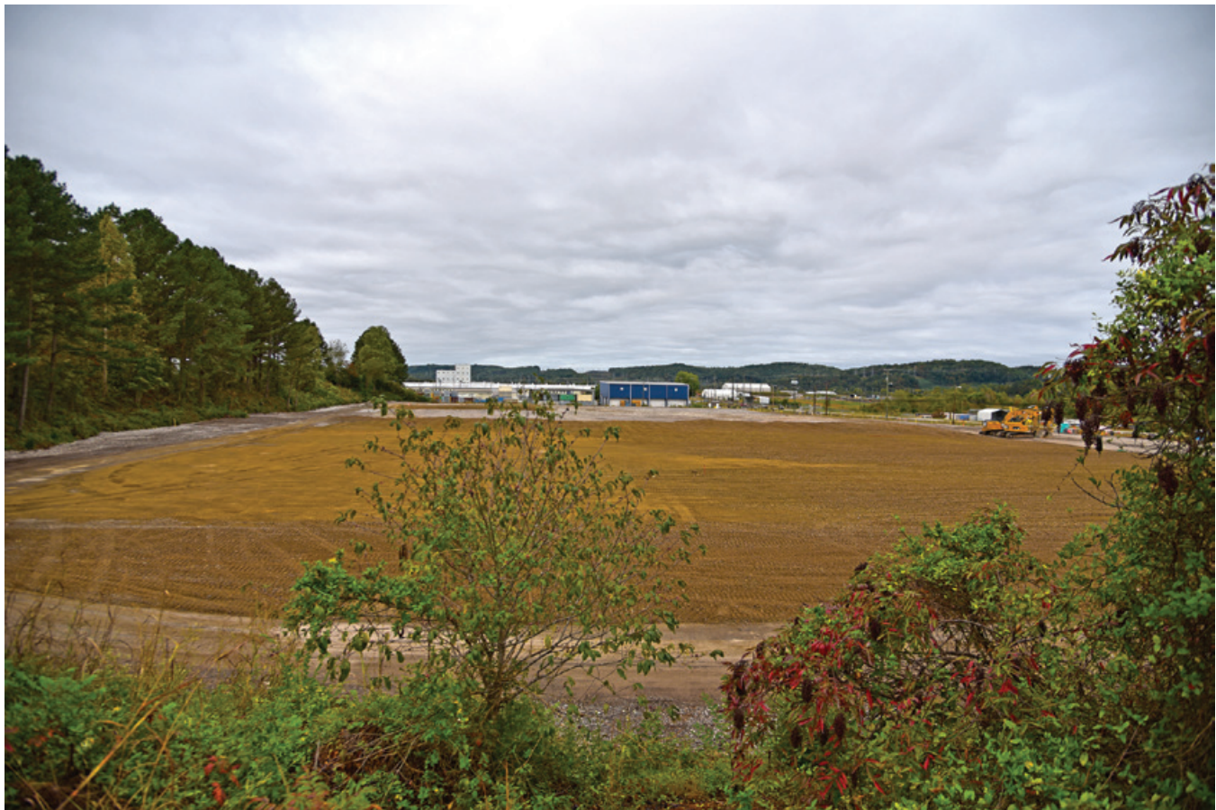
K-1037 site after demolition and slab removal
