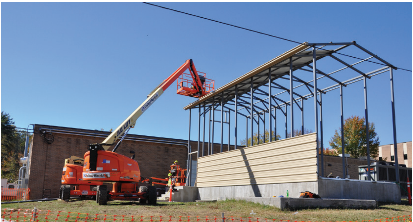
Workers construct housing for large tanks at the ORNL Aquatic Ecology Lab
