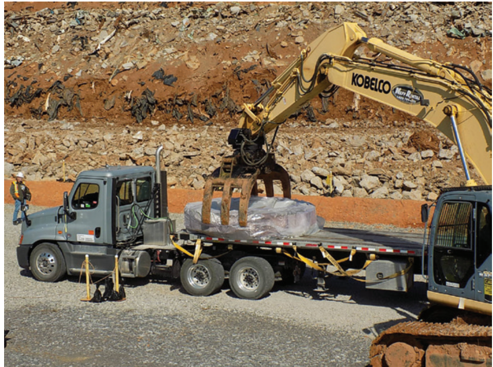
Receipt of oversized item at EMWMF
