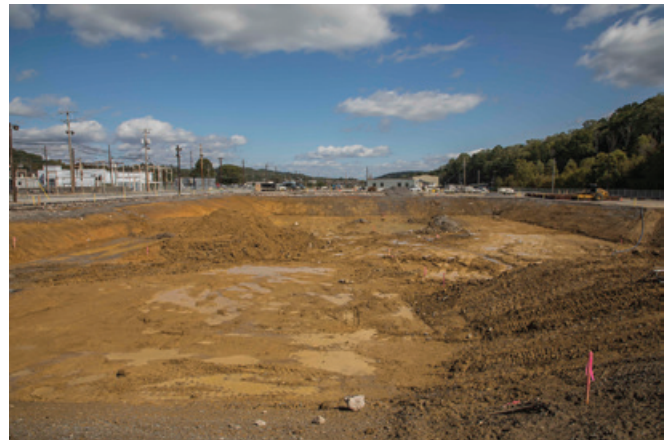
Excavation underway at the treatment facility area
