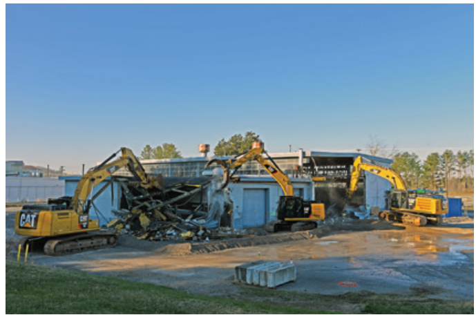
K-1414 Garage demolition
