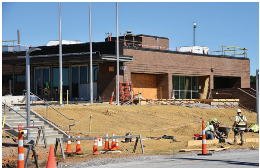
Workers are preparing walkways for the History Center
