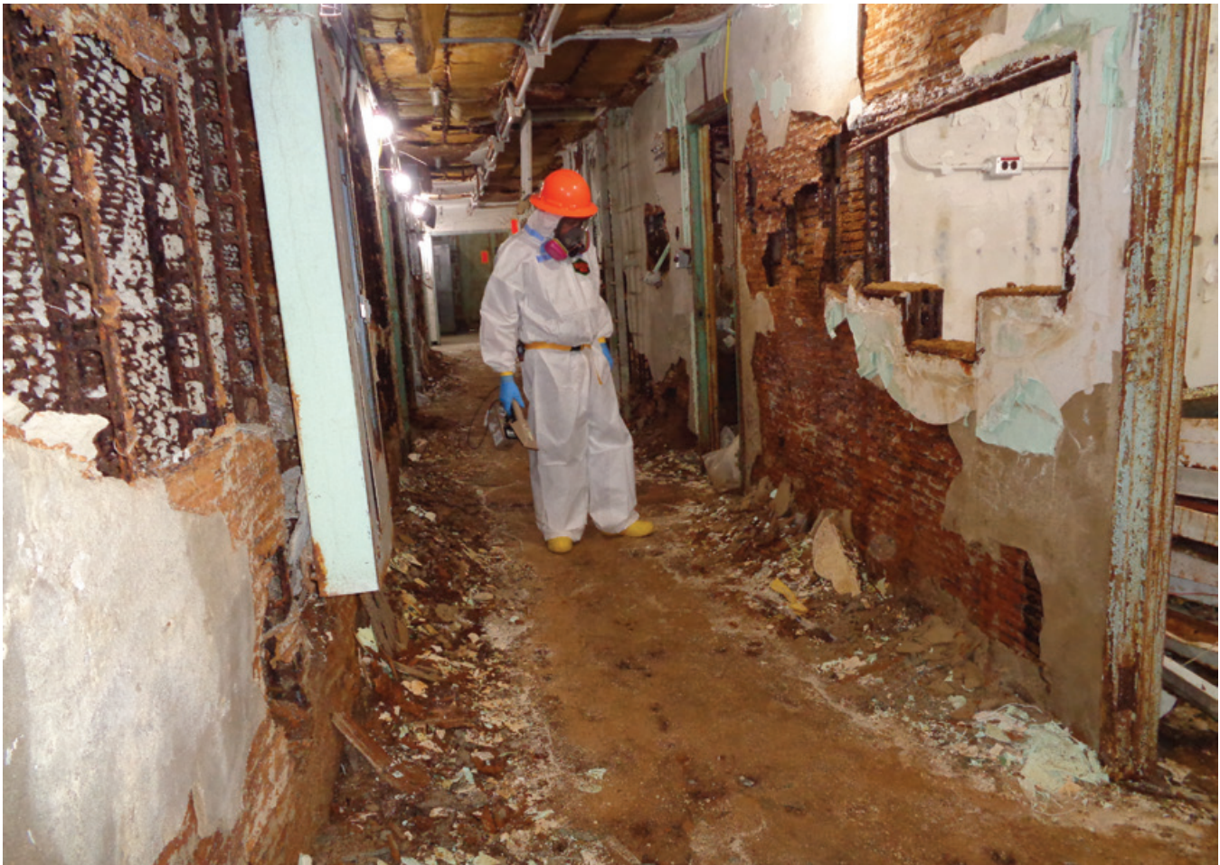
Workers perform characterization and asbestos abatement inside the Biology Complex to prepare the structures for demolition in 2020
