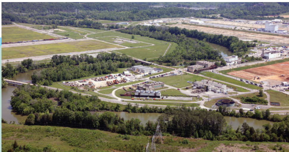
The Poplar Creek area before and after the process buildings were demolished
