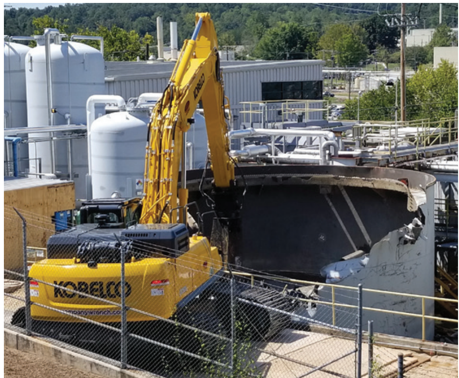
Workers are demolishing equipment at 3608 to make room for new equipment
