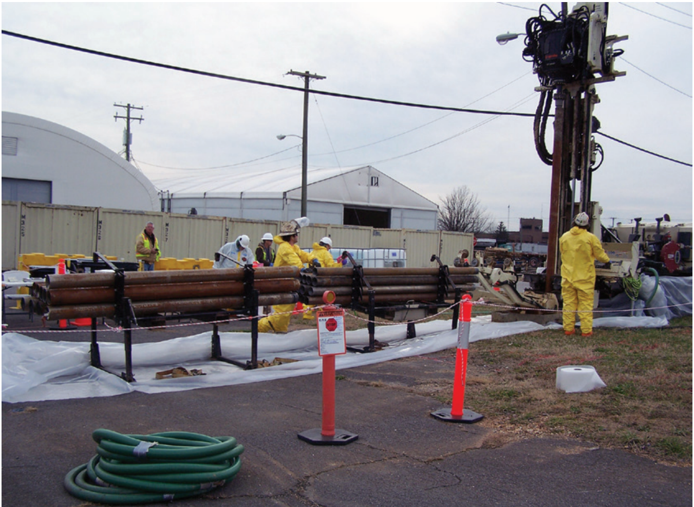
The Oak Ridge Reservation has an extensive network of monitoring wells that provide valuable groundwater data
