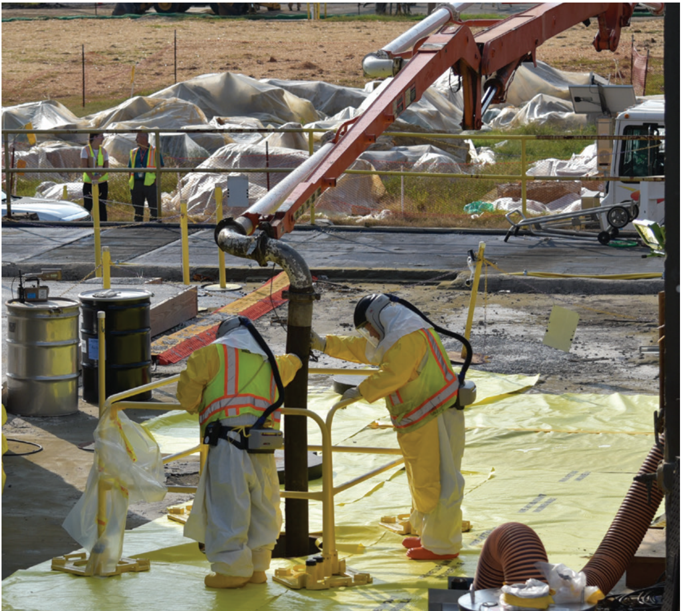
Workers grout the transfer tunnel at the 3026-D hot cell
