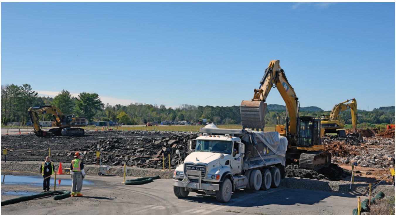
The slab removal at the K-29 site opens up more land for industrial development
