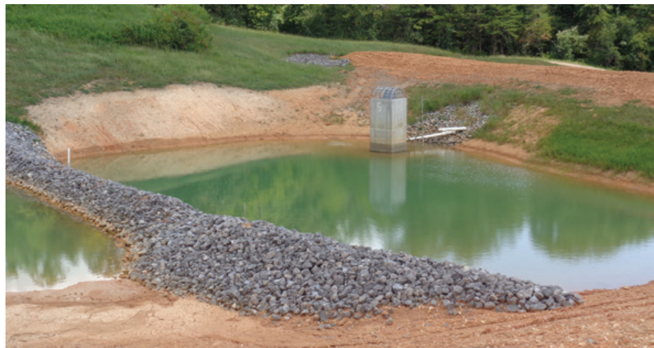
Erosion controls put in place at the Oak Ridge Reservation Landfills
