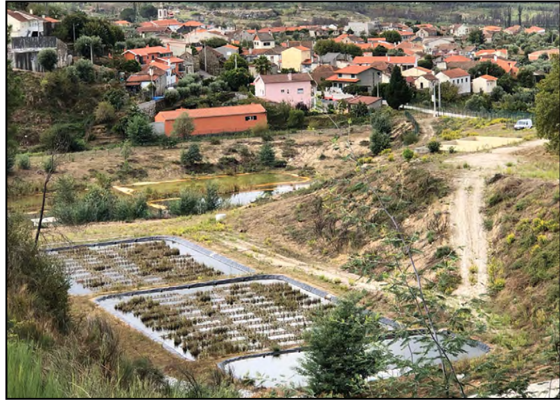
Cunha Baixa Old Mine in Portugal. Remediation technologies include active and passive wastewater treatment systems near a residential area.
