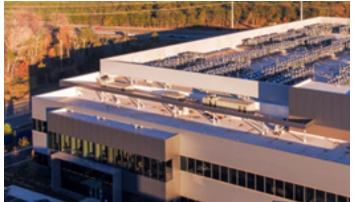
Figure 22. Better Buildings Data Center partners showcase the integration of various building energy efficiency technologies, including server rack blanking panels, LED lighting, separate computer room air handler (CRAH) aisles, and advanced metering utilizing data analytics and artificial intelligence to enable near-real-time system optimization. Image courtesy of the Better Buildings Initiative
