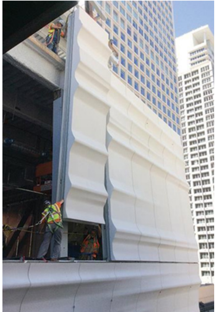
Figure 18. Installation of a fiber-reinforced polymer panel manufactured by Kreysler and Associates for the San Francisco Museum of Modern Art. Image courtesy of Kreysler and Associates
