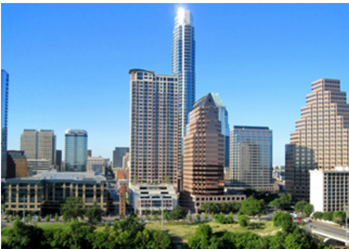
Figure 20. Commercial buildings represent over 90 billion square feet of floor space, a significant opportunity for reducing energy waste.
