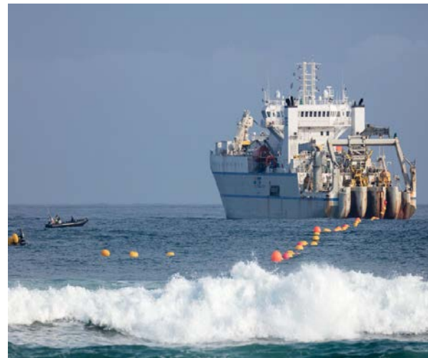
Subsea cable laying operations
