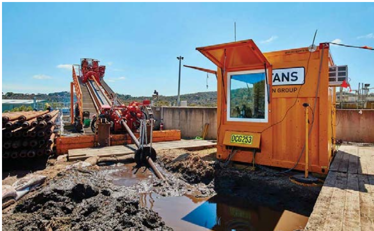
Horizontal directional drilling (HDD) operations
