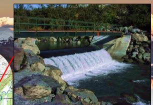
Power Creek Hydroelectric 6278kW (2 x 3124 kW) 25 kV transmission ties to Eyak Substation, Inflatable dam
