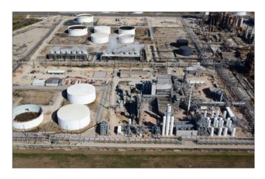
The ADM project started commercial operations on April 7, 2017 and has already achieved its full injection rate of 925,000 metric tons of  $\rm CO_2$  per year. As of August 2019, 1.32 million metric tons of  $\rm CO_2$  have been injected into the Mount Simon Sandstone saline reservoir.
