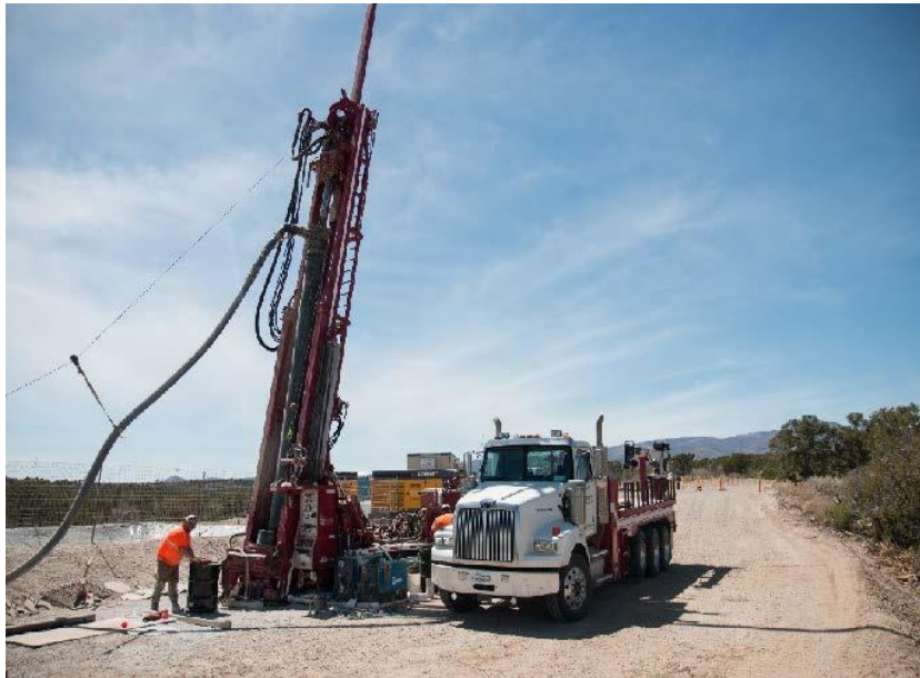
Angled drilling has enabled wells to be installed in locations that otherwise would not have been possible.
