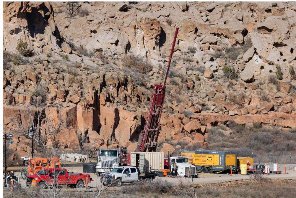
The monitoring well R-70 was installed in spring of 2019.
