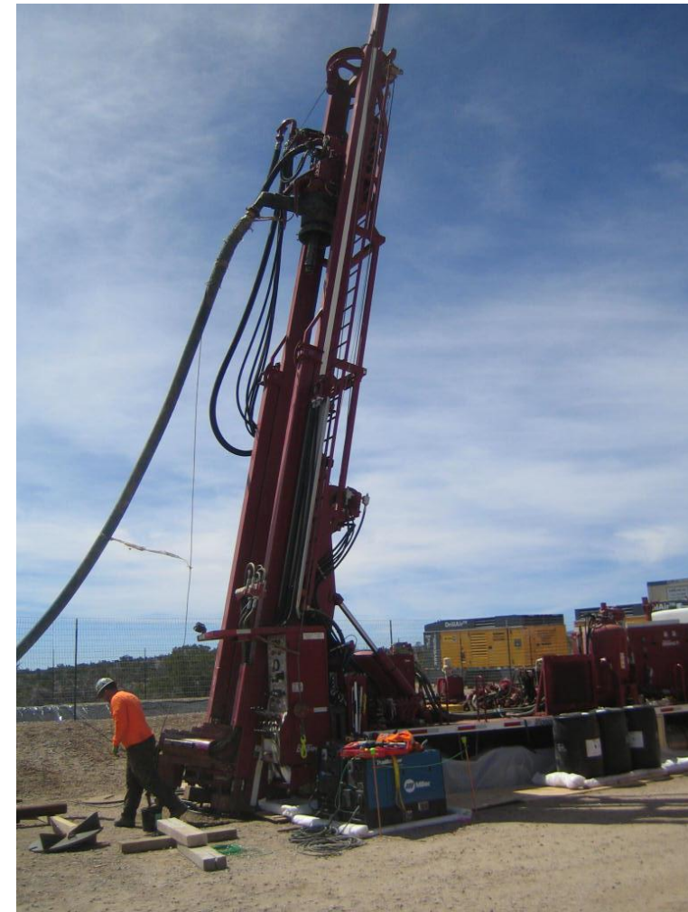
Angled drilling has enabled wells to be installed in locations that otherwise would not have been possible.
