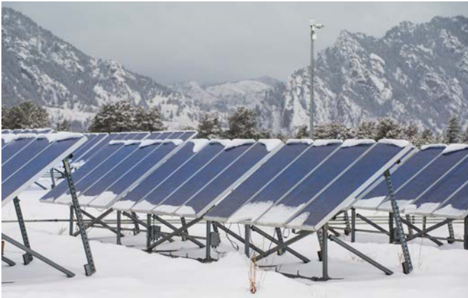
Snow melts off a photovoltaic array at the NWTC. Photo by Dennis Schroeder, NREL 54916
