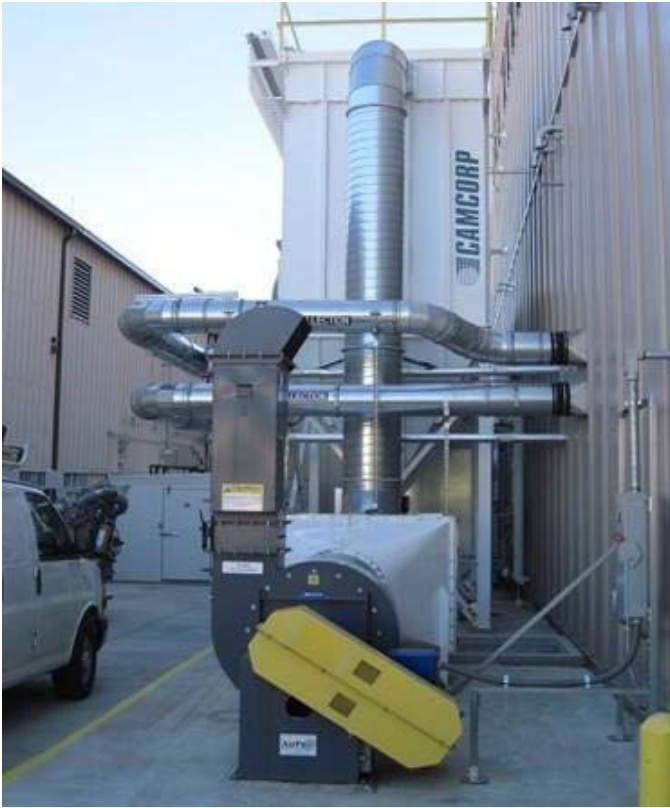
The particulate baghouse scrubber at the Integrated Biorefinery Research Facility removes particulate from exhaust air during pre-processing of biomass prior to experiments. Photo by Larry Durbin, NREL 56271
