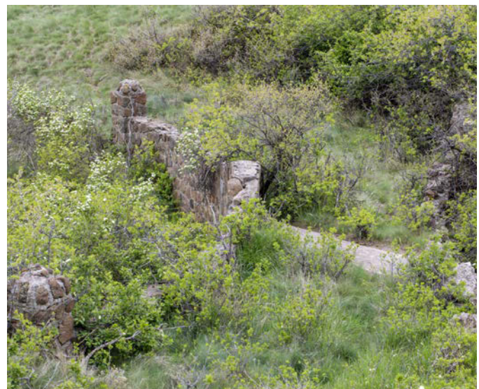
A stone bridge spanning a natural drainage channel at the STM site. The bridge, together with an open-air amphitheater, was constructed in 1935 and is listed on the National Register of Historic Places. Photo by Werner Slocum, NREL 56824
