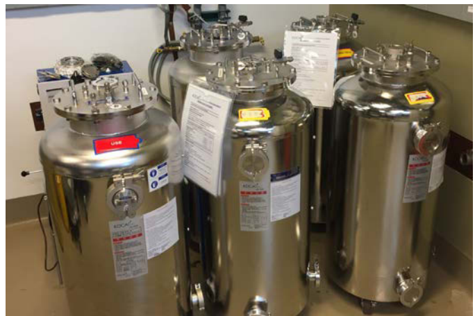
Point-of-use abatement canisters used to remove hazardous gases from the process exhaust during photovoltaic fabrication. Photo by Eric Schmitz, NREL 56941
