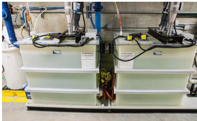
A waste neutralization system used to treat discharge from a solar cell etching research tool in the Science and Technology Facility at the STM site. Photo by Werner Slocum, NREL 55936
