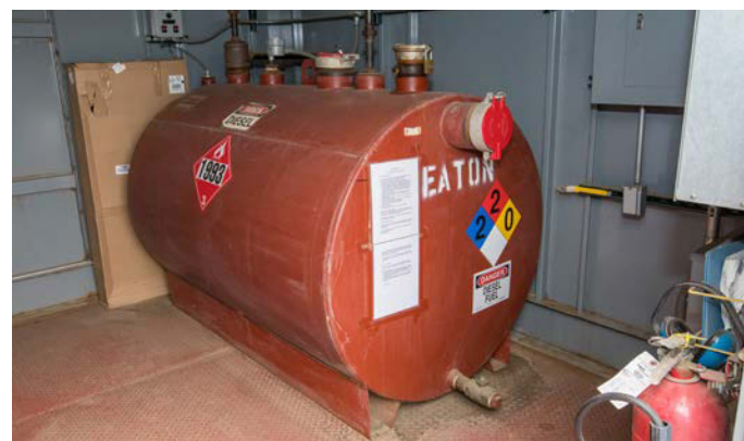
A diesel fuel tank is located inside the building that houses “Big Buck,” an emergency generator at the STM site. Photo by Werner Slocum, NREL 55987
