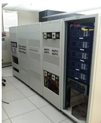
HTB Hardware room
