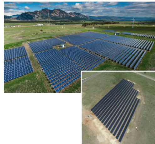
NREL-First Solar Project
