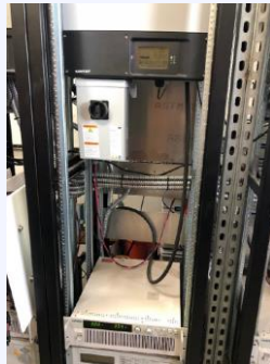
SolarEdge and SMA Inverters
