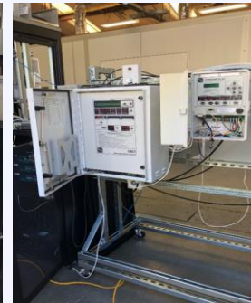
Cap Bank and Switch Controller
