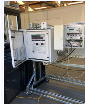
Cap Bank and Switch Controller
