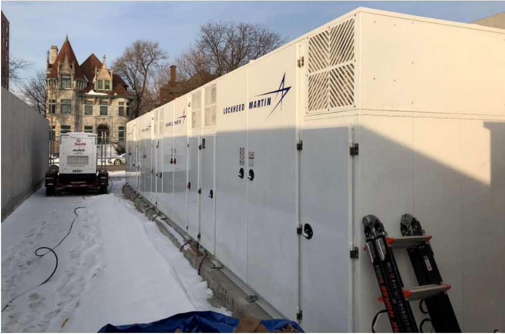
Battery Energy Storage Installation
