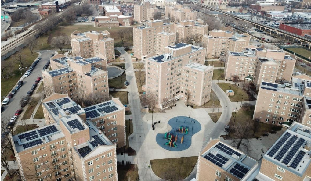
Solar PV Installation
